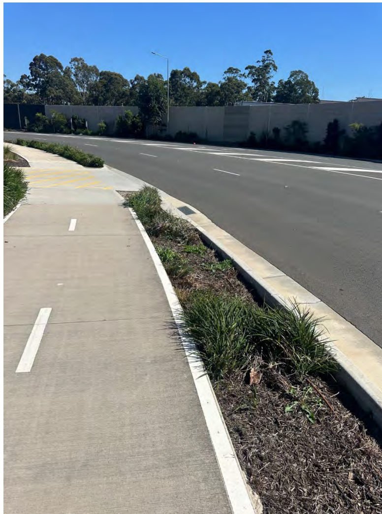
Figure 38 - Evidence of ground cover mortality at Warehouse N1 (09/04/2026).
