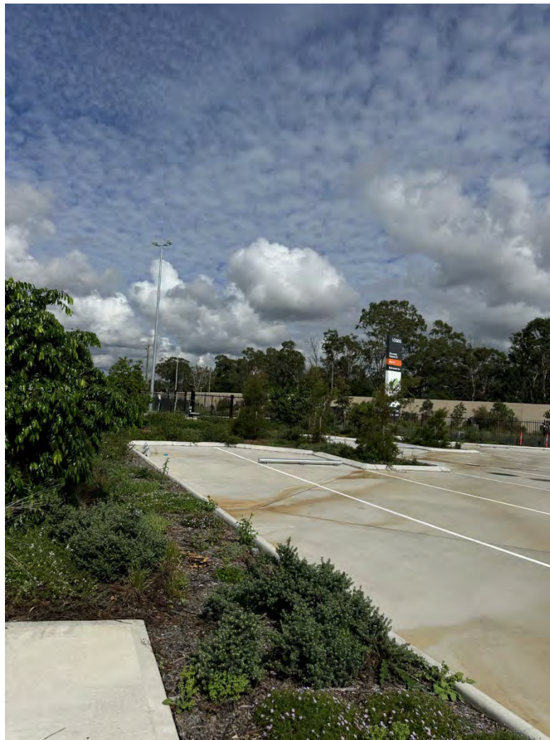
Figure 11 – Example of shade tree planting at Warehouse MoRDC (13/03/2025).
