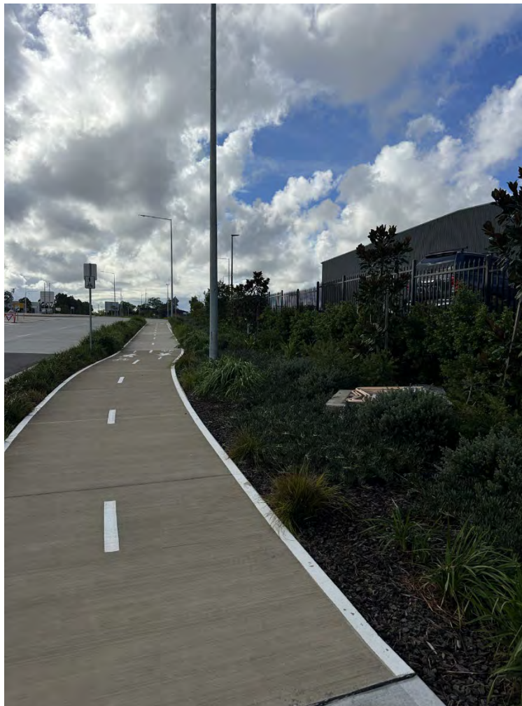
Figure 35 - Example of ground cover vegetation implemented in accordance with the UDDR. Subject example at is at Bapaume Road (13/03/2026).
