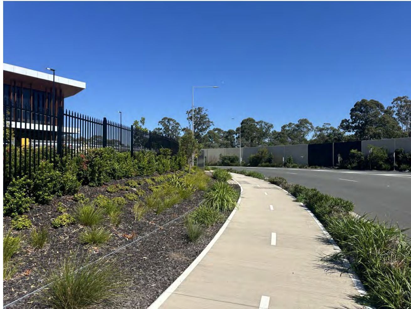
Figure 81 – Example of the 5m setback from the internal road to warehouse carparking. Subject example is at Warehouse N1 (09/04/2026).
