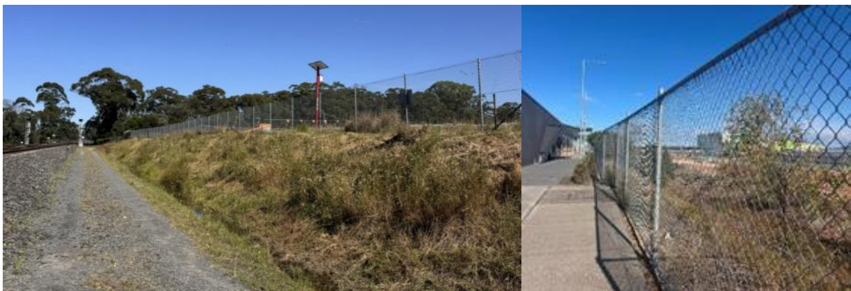
Plate 3-1. Left: Soft batters in the Rail Link corridor following weed removal works by Toolijooa, native grasses ( Themeda triandra and Dichanthium sp. ) are growing substantially with weed growth suppressed particularly in the areas immediately adjacent to the BioBank Site. Right: at the IMEX building and adjacent drainage infrastructure Acacia falcata (Hickory Wattle) continue to grow unimpeded by weeds.
