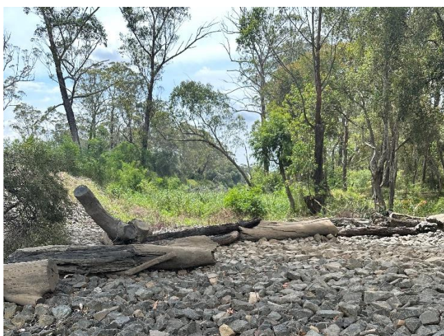
Plate 4-1. Large logs and piles, of course, woody debris placed to facilitate movement of fauna across ballast at Georges River beneath the rail link bridge
