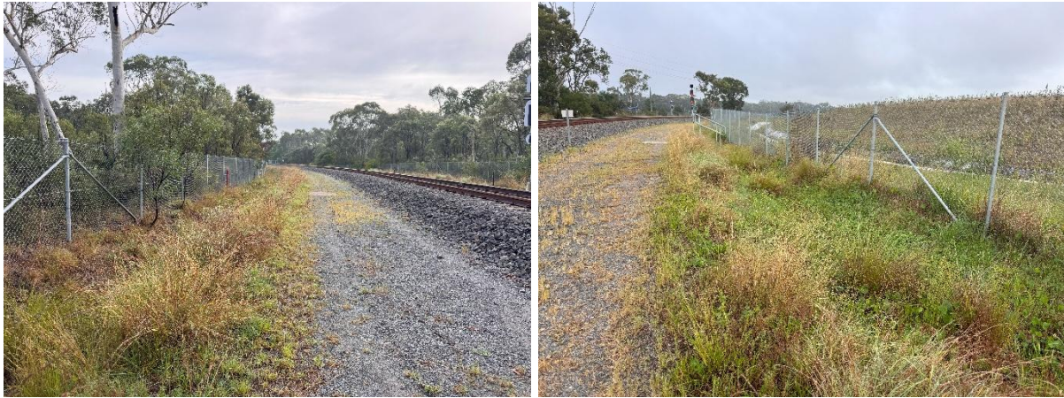
Plate 3-2. Soft batters in the Rail Link corridor following weed removal works by Toolijooa.
