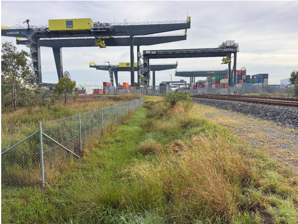
Plate 3-1 Photographs captured during the February 2025 inspection showing low weed cover in the Rail Link. Native grasses have begun heavily colonising the on soft batters on either side of the rail line.
