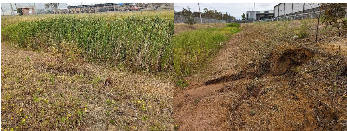
Plate 2. Observation of native plant damage and erosion in drainage basins.
