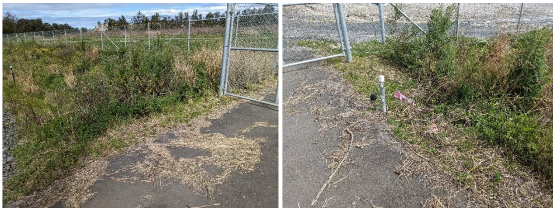
Plate 4 Evidence of slashing at the western side of the rail link corridor
