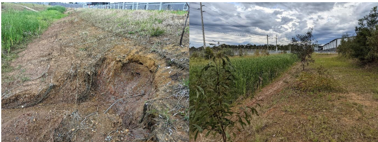
Plate 2. Observation of native plant damage and erosion in drainage basins. Observations were also present in the August 2022 survey.
