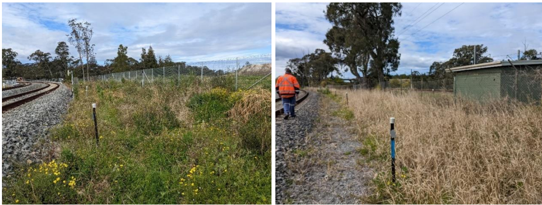
Plate 6. Exotic species, Rhodes Grass and Fireweed continue colonising remediating soft batters within the Rail Link corridor
