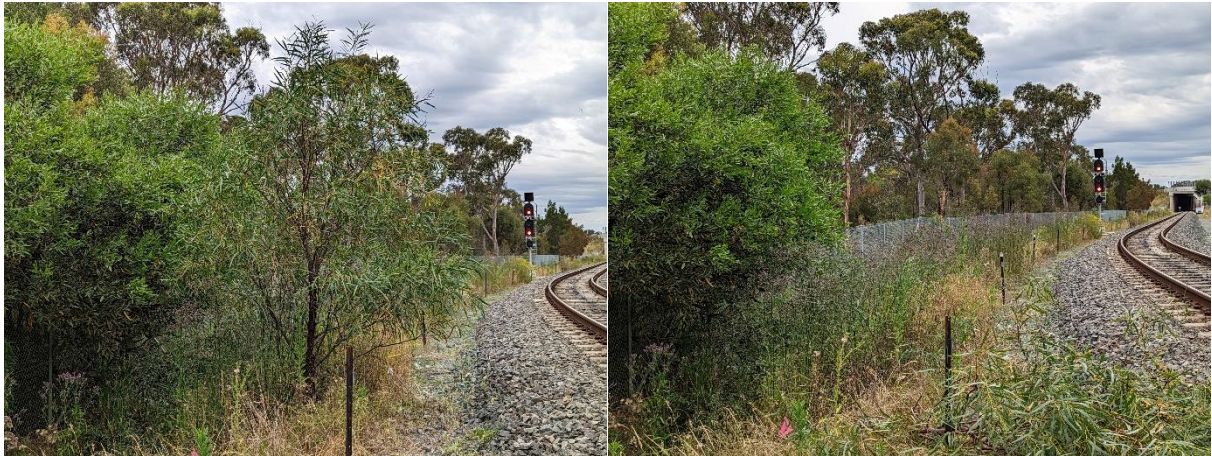
Plate 6 Instance of Golden Wreath Wattle removal due to location of tree impeding vision of traffic signal
