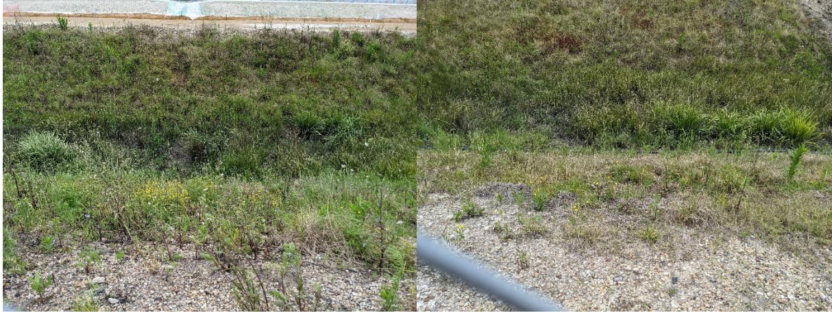
Plate 3 Fireweed growing on soft batters of the northeast trunk drainage system.
