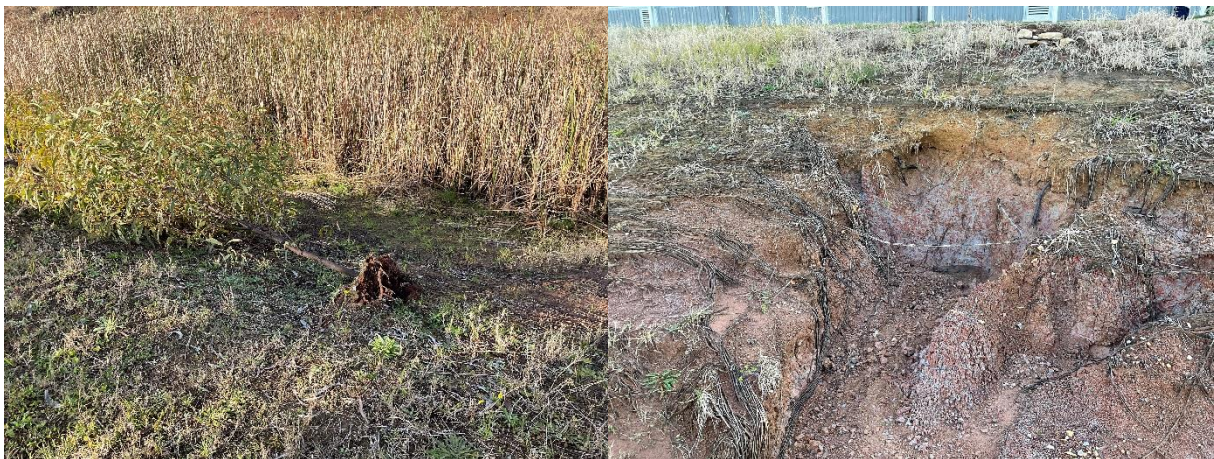
Plate 2. New observation of native plant damage and erosion in drainage basins
