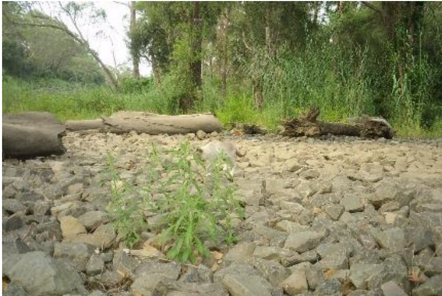
Plate 4-1. Large logs and piles, of course, woody debris placed to facilitate movement of fauna across ballast at Georges River beneath the rail link bridge
