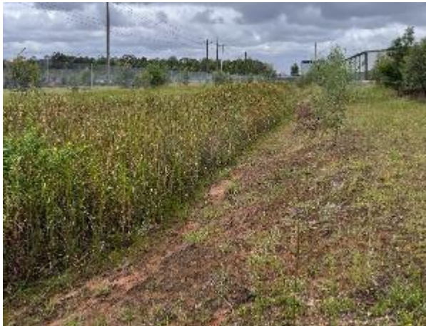
Plate 3-1 Photographs captured during the February 2023 inspection showing low weed cover and established native plants observed on soft batters surrounding the basins and drainage channel at the north-eastern extent of the operation facility
