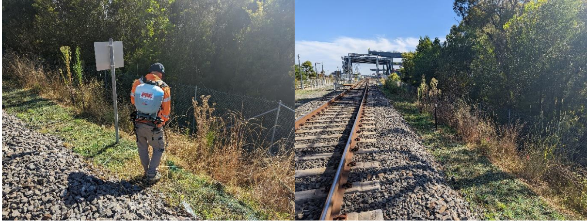
Plate 3-2. P&E Service undertaking weed control works within the Rail Link
