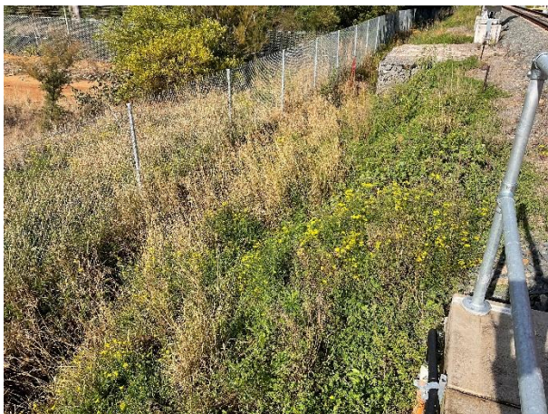
Plate 4. Exotic species, Rhodes Grass and Fireweed, continue colonising remediated soft batters within the Rail Link corridor
