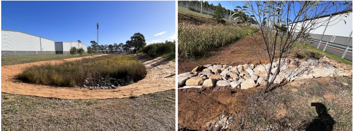
Plate 2. Rectification measures for instances of erosion in the drainage basin (left), and around the stormwater outlet (right).
