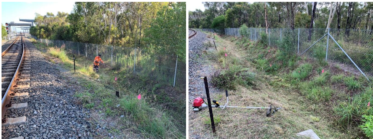
Site photograph 3. Soft batters in the Rail Link corridor following weed removal works by P&E Services. Note the reduced cover of exotic species and retention of native species next to pink survey flags.
