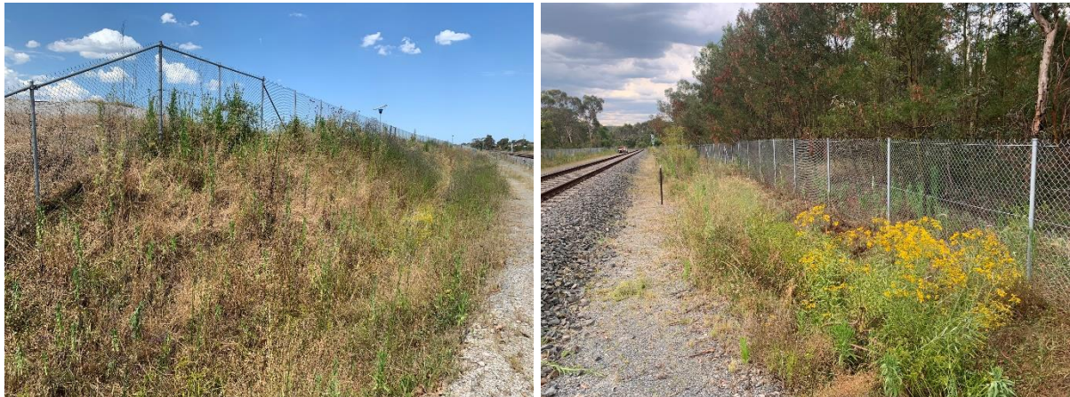
Site photograph 2. Soft batters in the Rail Link corridor prior to weed removal works by P&E Services. Note the high cover and biomass of weed species
