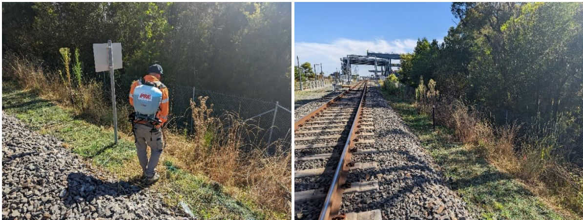
Site photograph 1. P&E Services employee applying herbicide to plants on gravel and ballast areas using a backpack sprayer.
