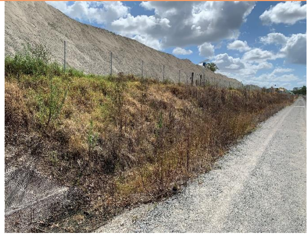
Majority of weed treated with herbicide along the northern batters of the Rail Link
