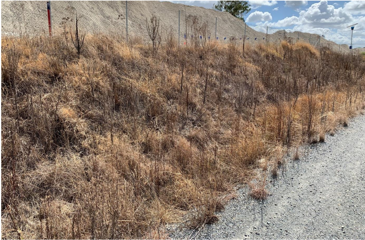
Plate 2. Dead weeds along soft batters in Rail Link following spraying with herbicide
