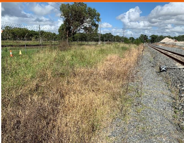
Partial treatment of weeds with herbicide on the southern side of Rail Link
