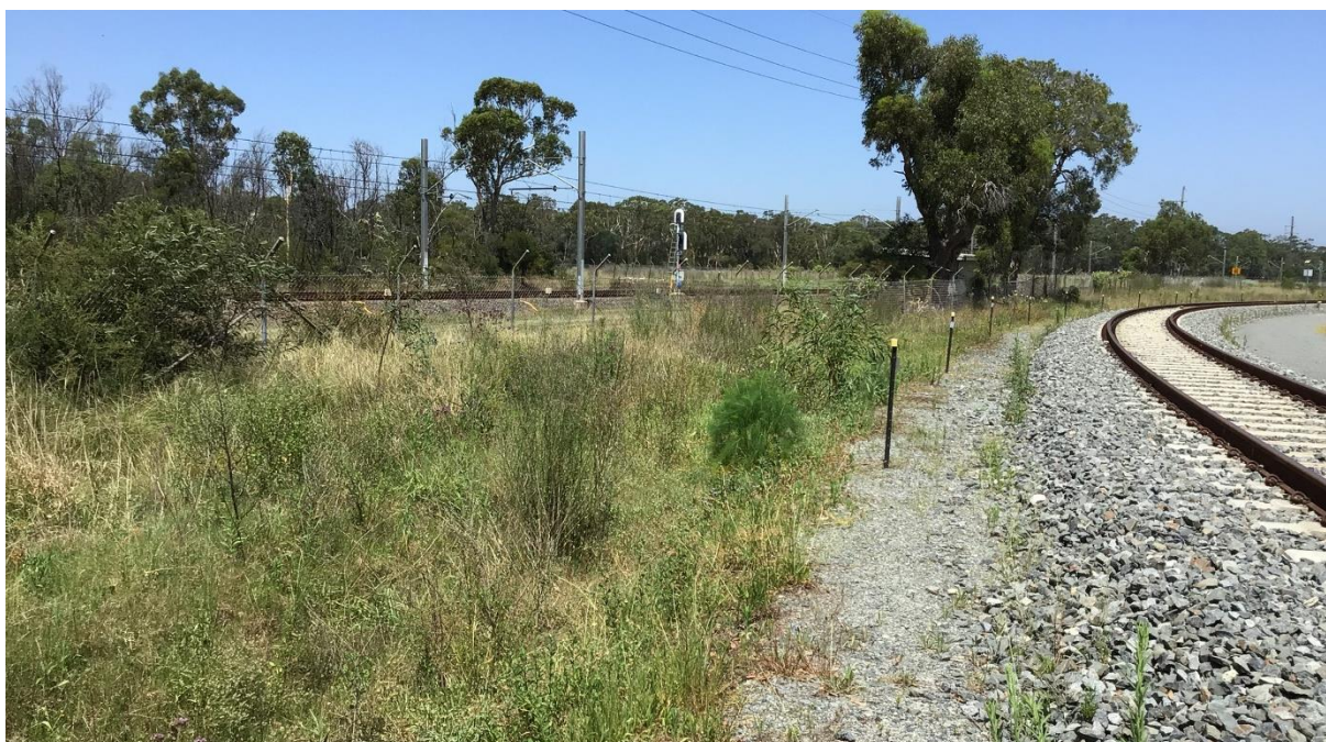
Plate 4. Weeds dominating non-remediated areas within the Rail Link
