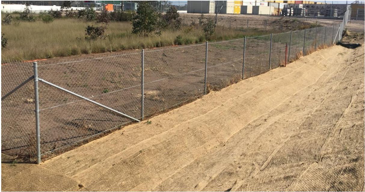
Plate 2. Soft batters being remediated through removal of weeds and stabilisation with coir mesh
