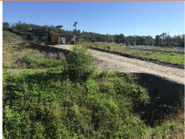
Environmental weeds colonising undeveloped lands at the western extent of the Rail Link.
