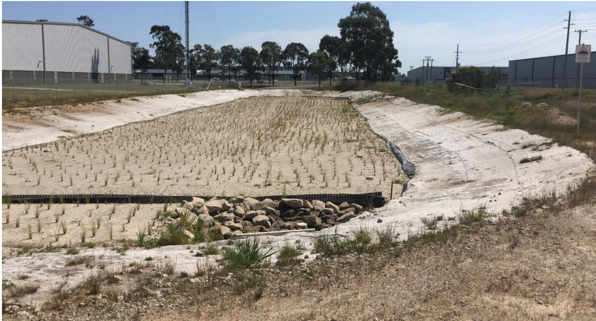
Plate 1. Drainage swale/retention basin in north eastern corner of operational area at risk of weed infiltration
