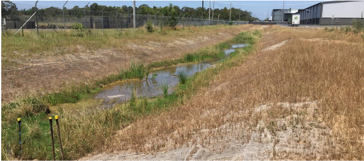
Plate 2. Senescing Secale cereale (Cereal Rye) on soft batters of drainage swale; increasing susceptibility of area to invasion by herbaceous weeds and aggressive invasive grasses.
