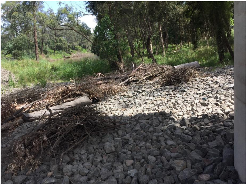
Plate 6. Large logs and piles of coarse woody debris placed to facilitate movement of fauna across ballast
