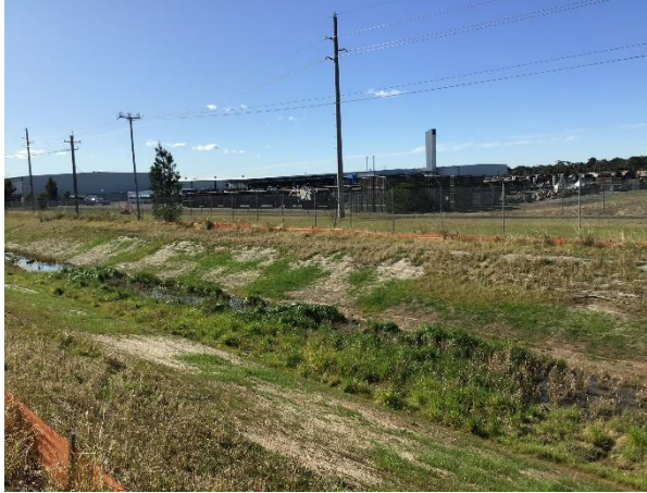
Slashing of exotic vegetation within the stormwater channel in the operational area.
