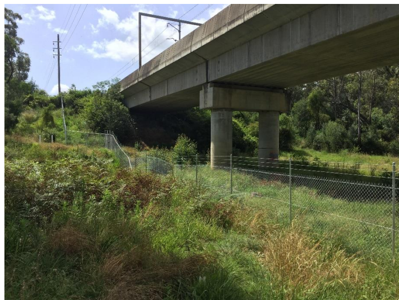
Plate 7. Newly erected cyclone fence at the southern extent of the management site
