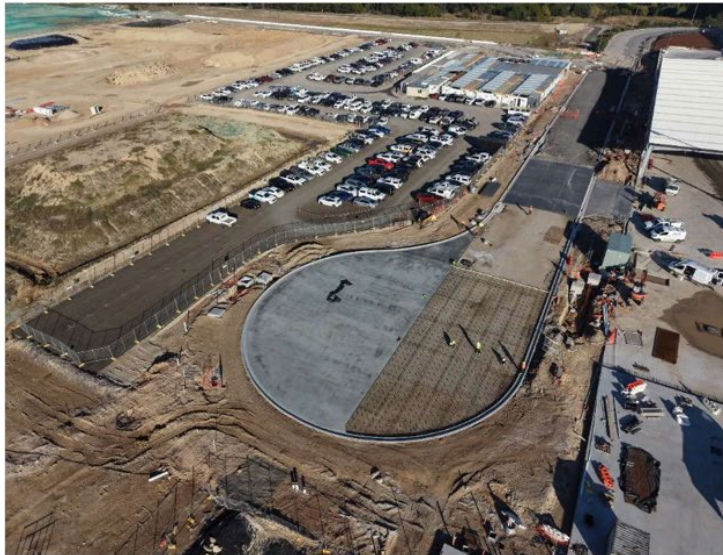
Figure 3: Bushmaster Ave Progress
