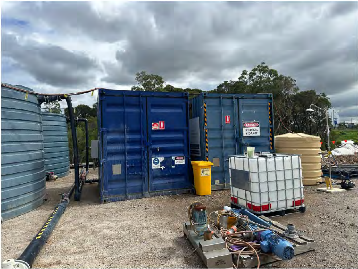
Photo 6: Chemical storage container and spill kit
