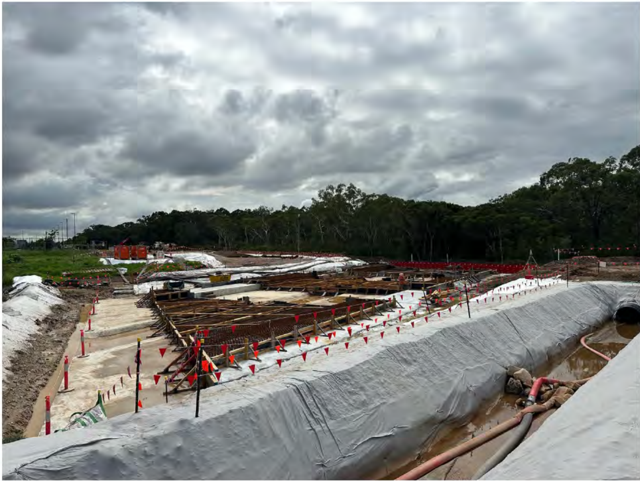
Photo 7: Geofabric lined clean water drain
