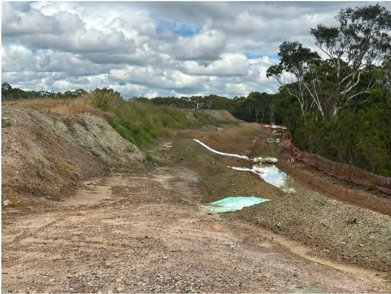
Photo 8: Stabilised batter and perimeter drain
