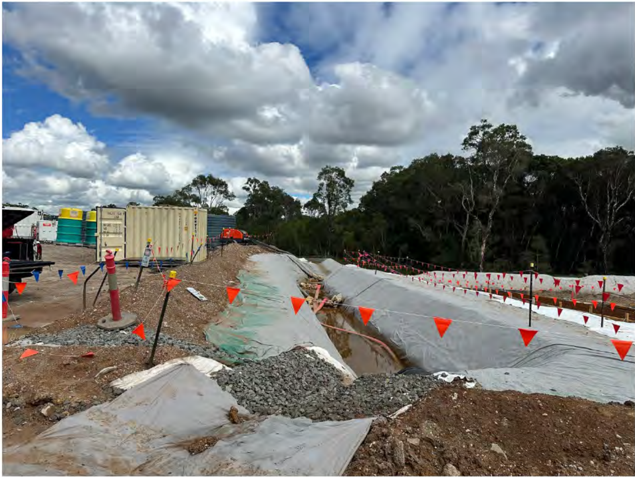
Photo 13: Geofabric lined drain
