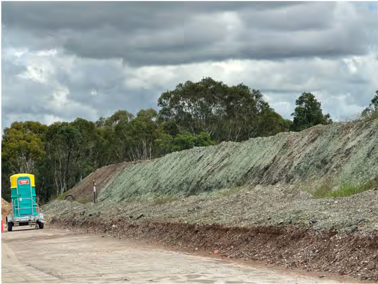
Photo 9: Polymer stabilised batter
