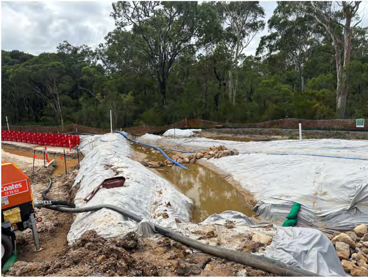
Photo 12: Geofabric lined drain
