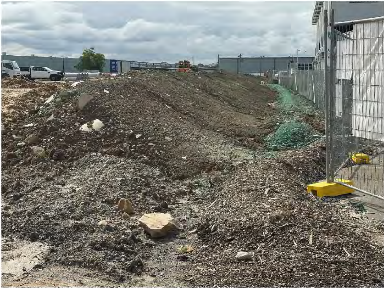
Photo 4: Shaped batter and stabilised bund
