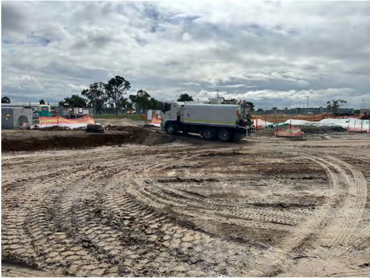
Photo 2: Water cart for dust suppression
