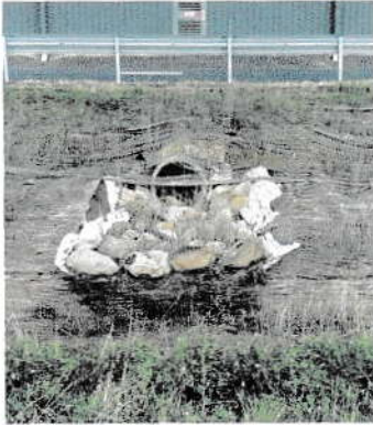
SW - 1 DISCHARGE OUTLETS AND CULVERTS NEED REPAIR EROSION OCCURRING AROUND ROCK CHUTE AND PIPE DUE TO NO HEAD WALL OR CULVERT.
