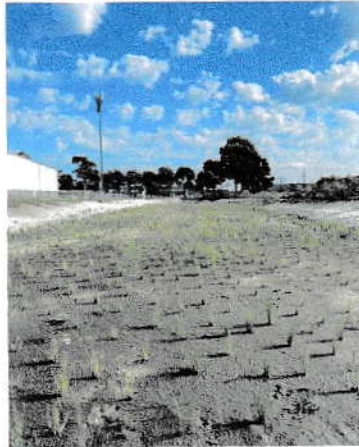
OSD-09 - WEEDING OF THE DETENTION BASIN, HAND REMOVAL AND SPOT HERBICIDE SPRAYING. INFILL PLANTING IS REQUIRED TO REPLACE FAILURE AREAS TO ENSURE CORRECT FUNCTION OF THE SYSTEM. INSTALL (100) UNITS OF REEDS AND SEDGES TO FILL IN GAP AREAS.
