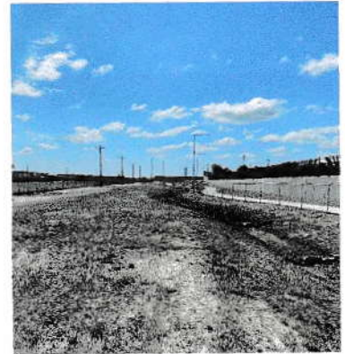
SWALE - INSPECTED AND RUBBISH REMOVAL
