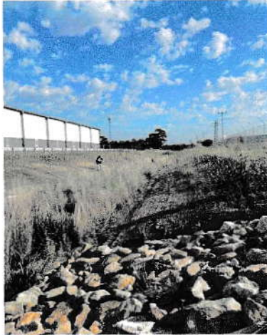
SW- 1 SPOT SPRAYING TARGETED WEED CONTROL, GRASSY SWALE BANKS AND FENCE LINE REQUIRE BRUSHCUTTING ON NEXT VISIT
