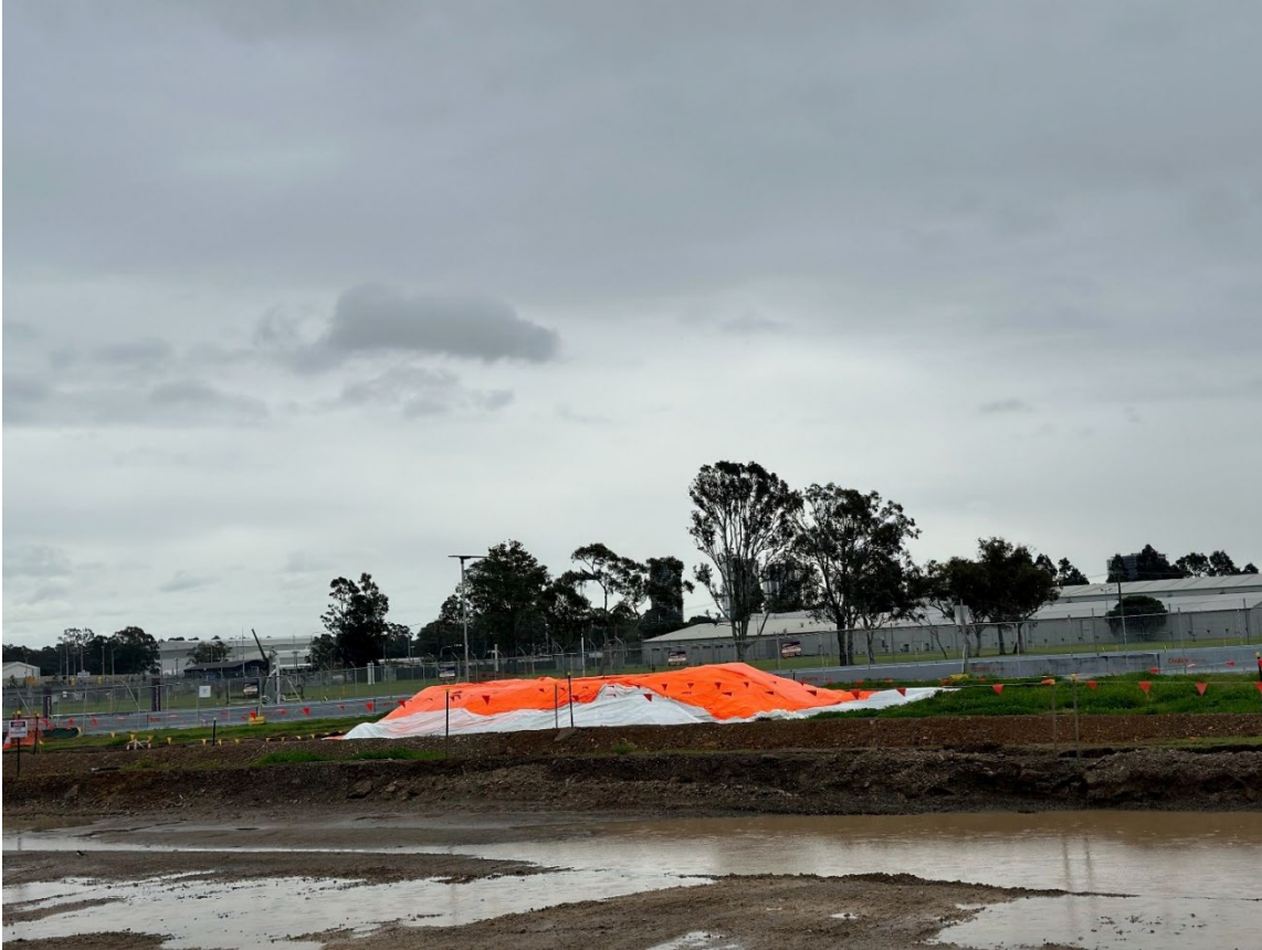
Photo 9: Covered asbestos soil stockpile
