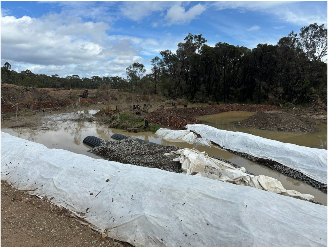
Photo 20: Anzac Creek protection measures and temporary diversion
