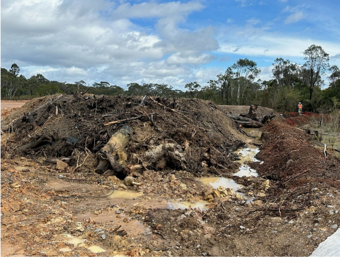
Photo 5: Timber mulch re-used for sediment controls
