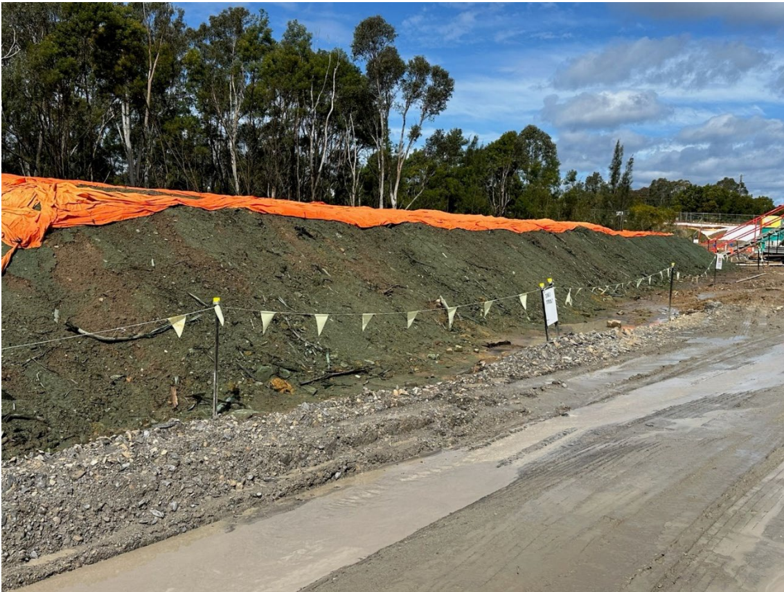
Photo 15: Polymer Stabilised batter
