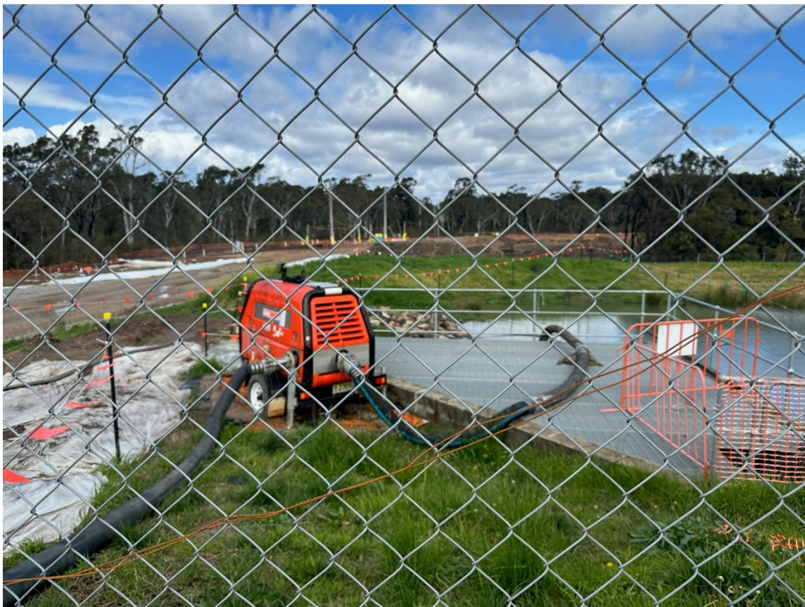
Photo 18: Clean water diversion pump (upstream inlet)
