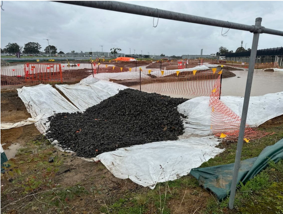
Photo 11: Sediment basin with rock overflow
