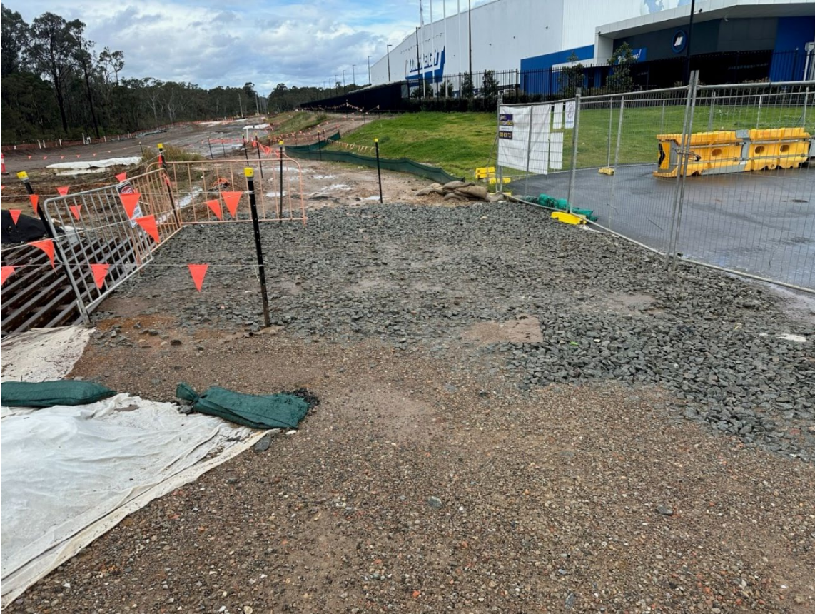
Photo 7: Stabilised site access and vehicle shaker grid
