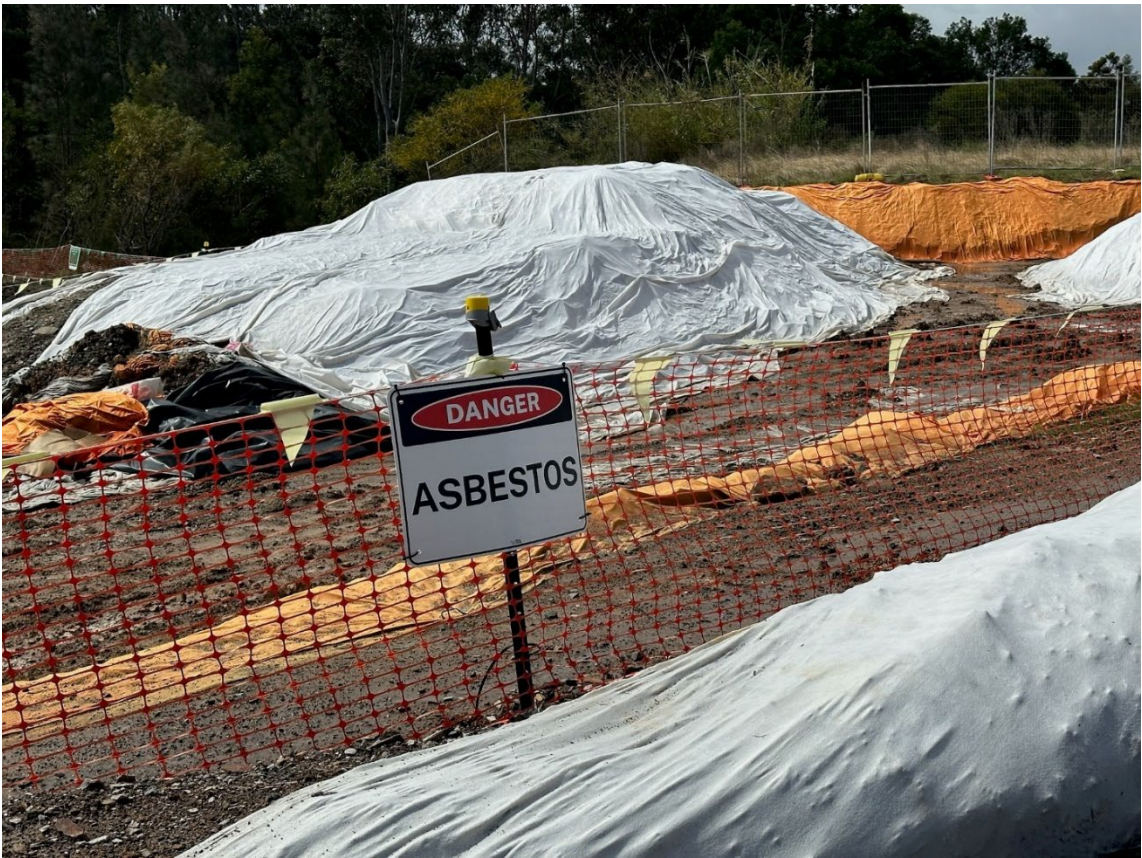
Photo 10: Covered asbestos soil stockpile and advisory signage
