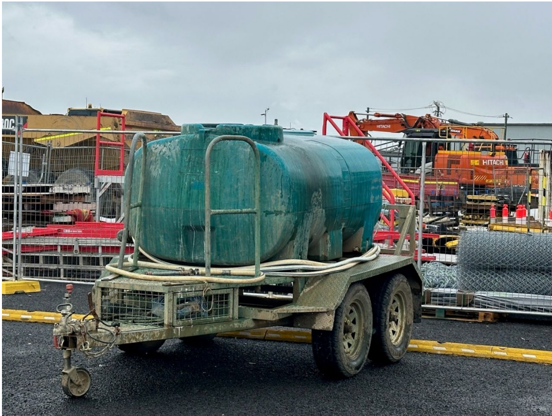
Photo 13: Mobile polymer trailer used for stabilisation of exposed areas
