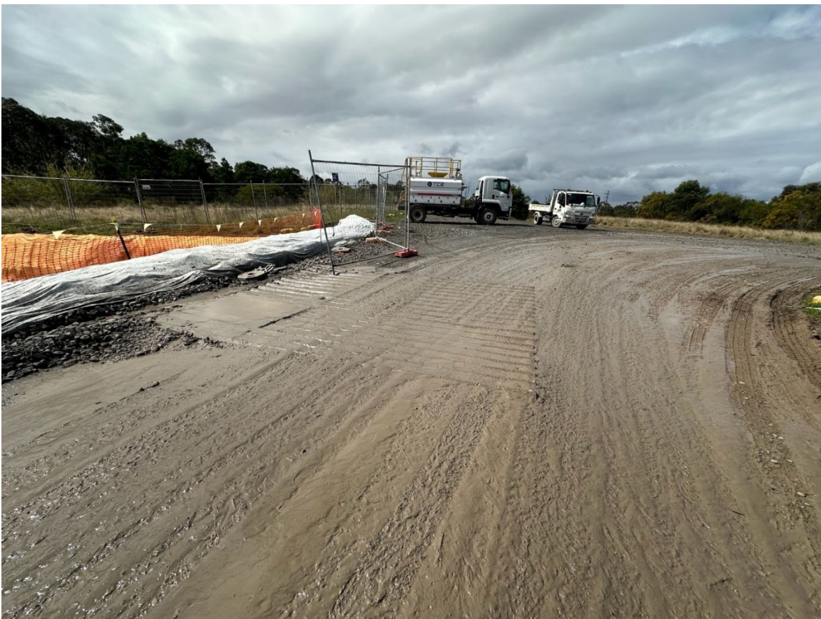
Photo 8: Rumble grid requiring clean out
