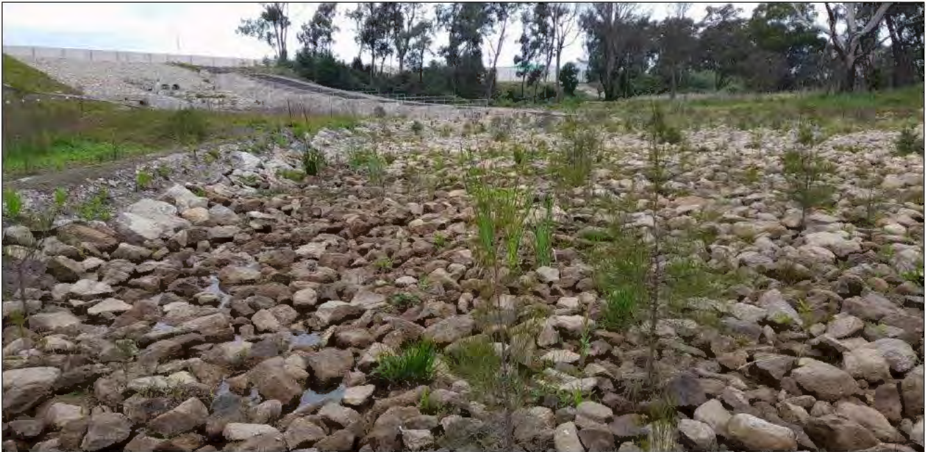
Site image: Outlet retention basin 5 MPW (Apical image 09 th October 2024)
