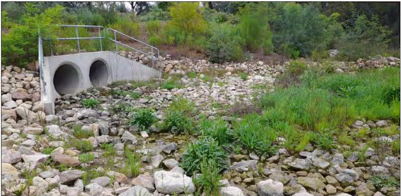
Site image: retention basin 6 MPW (Apical image October 2024)
