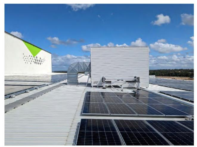
Figure 11 Example of what a roof looks like when it has been designed to include low albedo material. Subject example is on MoNDC where confirmation of low albedo material being used according to design will be confirmed in a future report.
