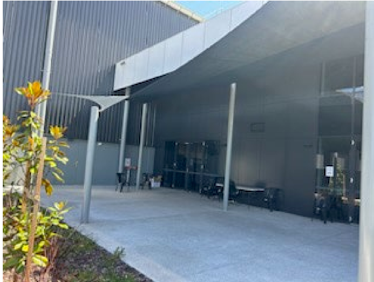
Figure B61 – 3 Outdoor break areas at warehouse N2
