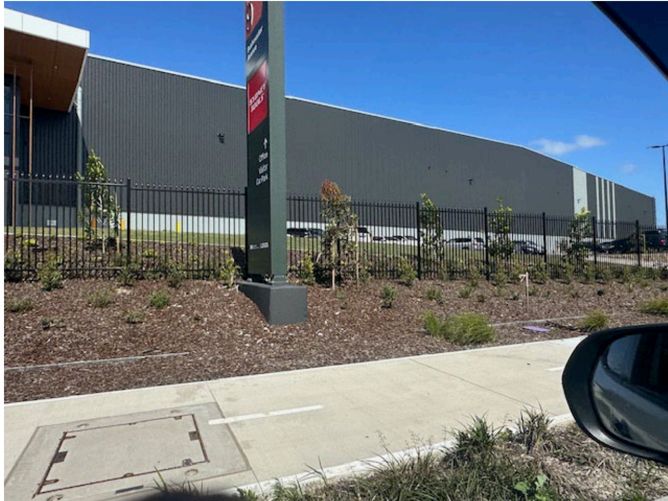
Figure B48 - 15 Low albedo material pavement
