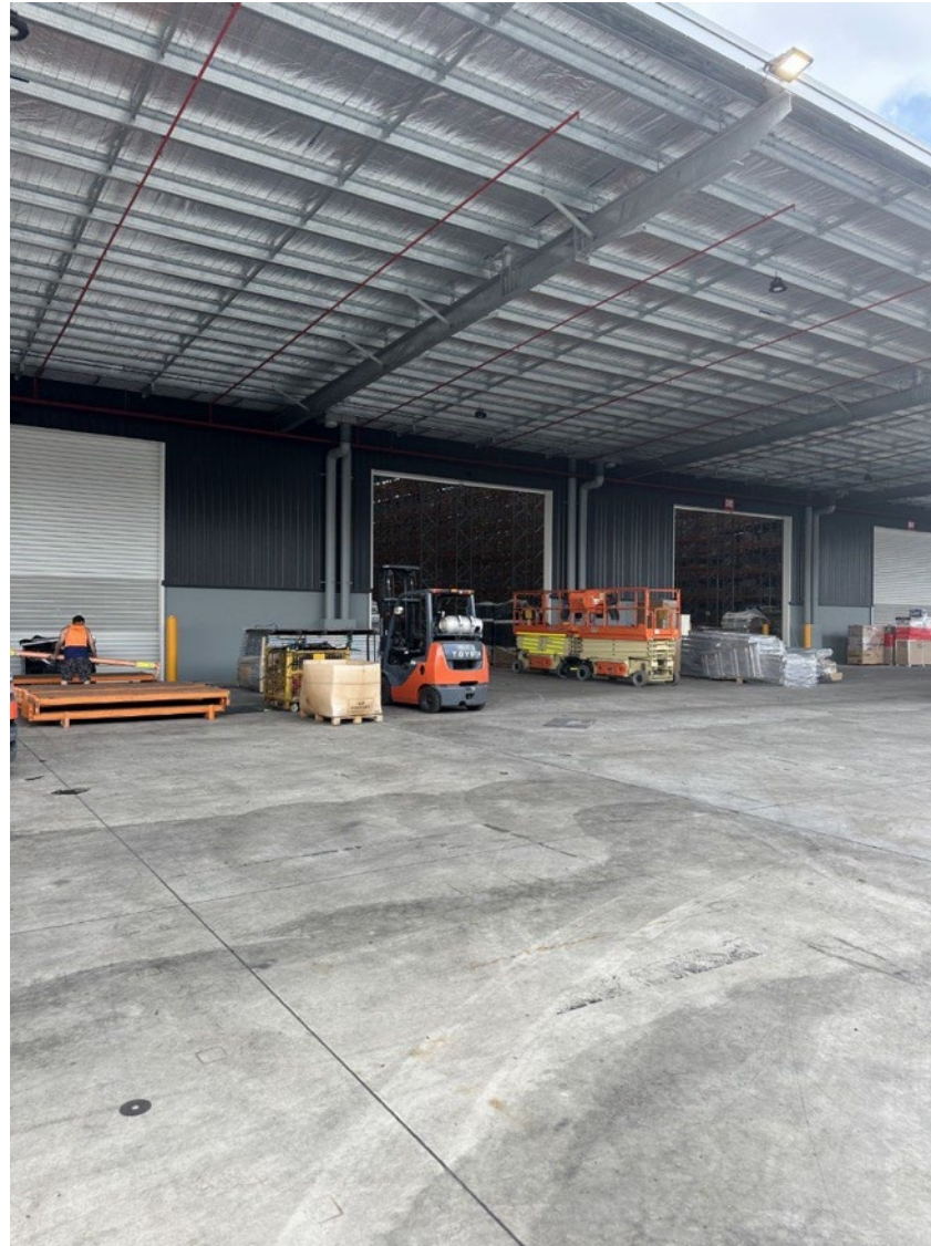
Figure B49 - 5 Awning and roller doors that can be used for cross ventilation at warehouse N2
