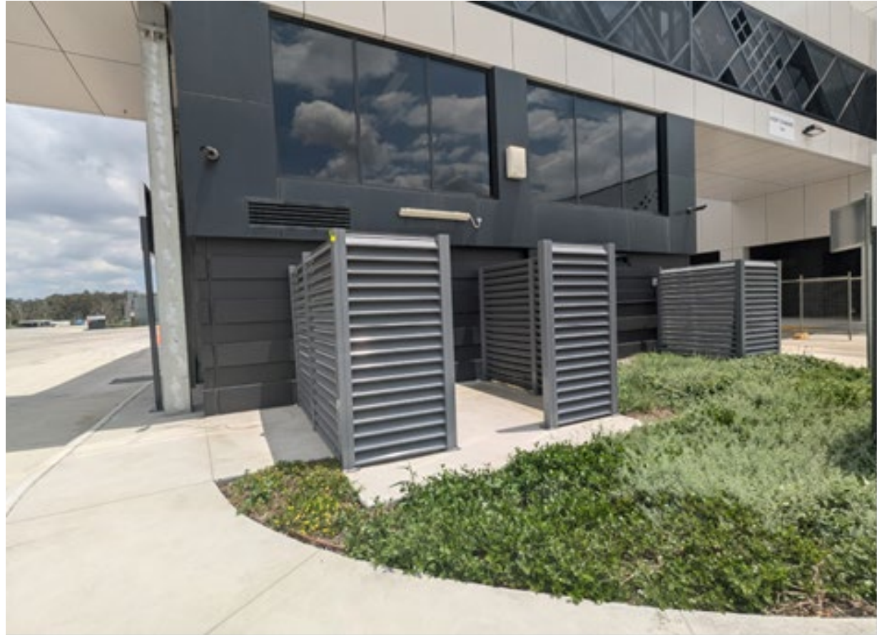
Figure 71 - 3 Outside screened area at warehouse JR and JN for storage.
