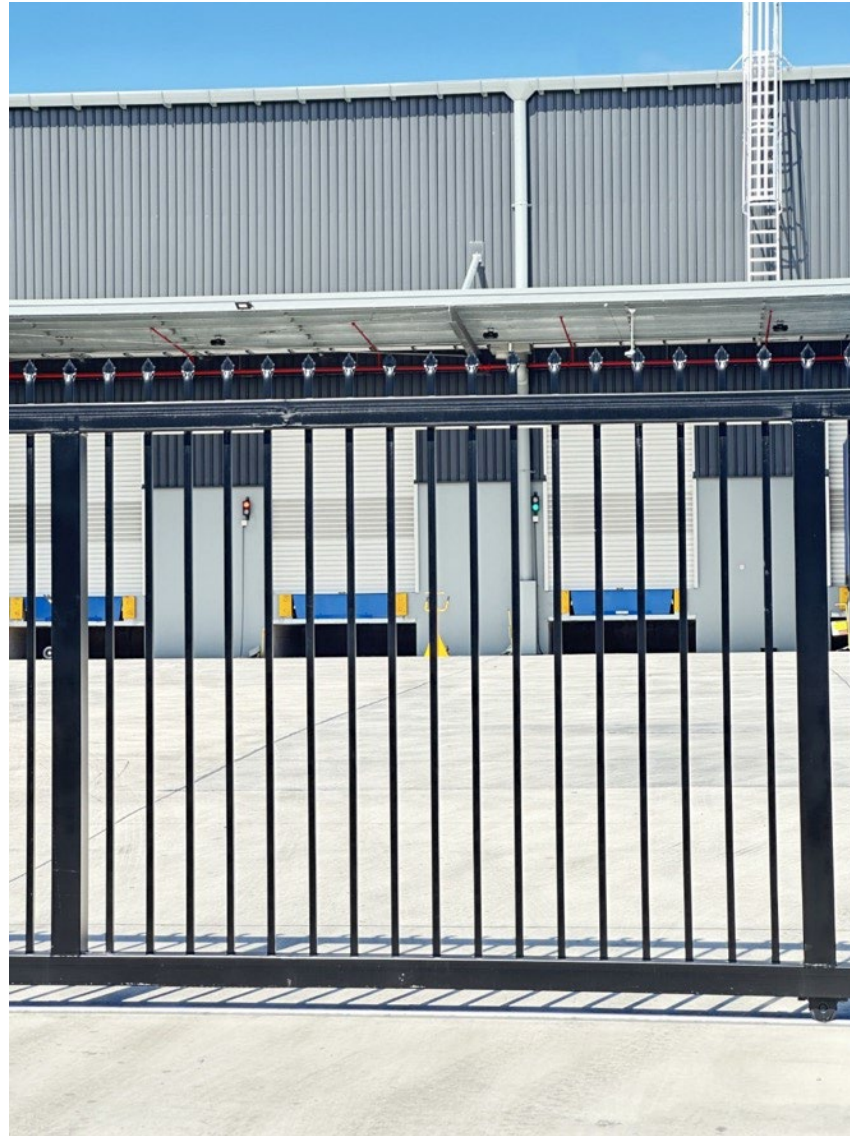
Figure B49 - 6 Roller doors that can be used for cross ventilation at warehouse N1
