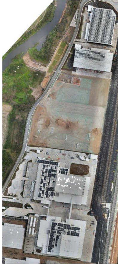
Figure B49 - 10 Aerial image showing open space between warehouses
