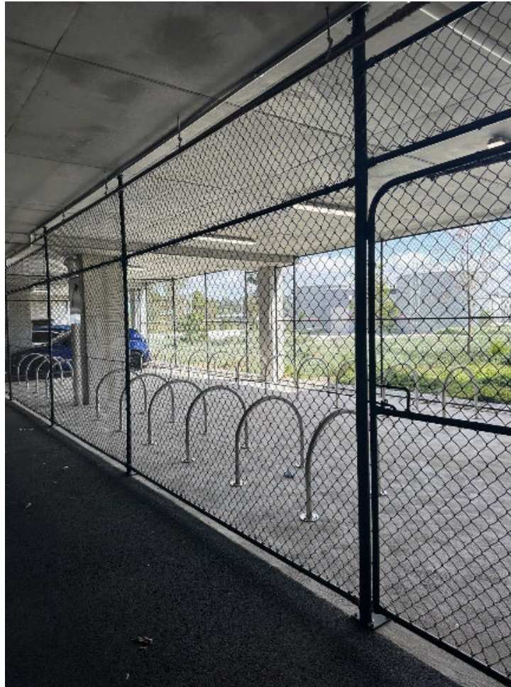
Figure B62 - 1 Secure bicycle parking located at warehouse JN
