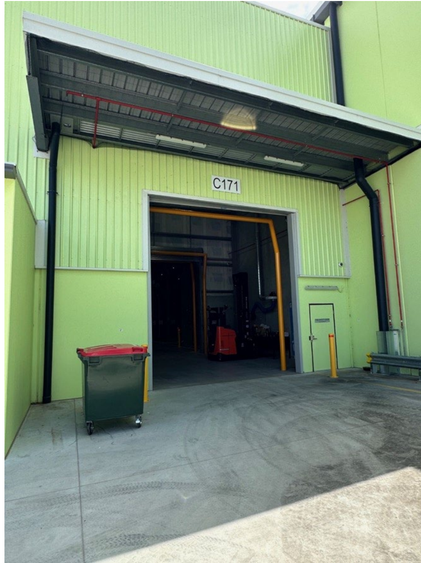
Figure B49 - 4 Completed awning and cross ventilation at warehouse JN
