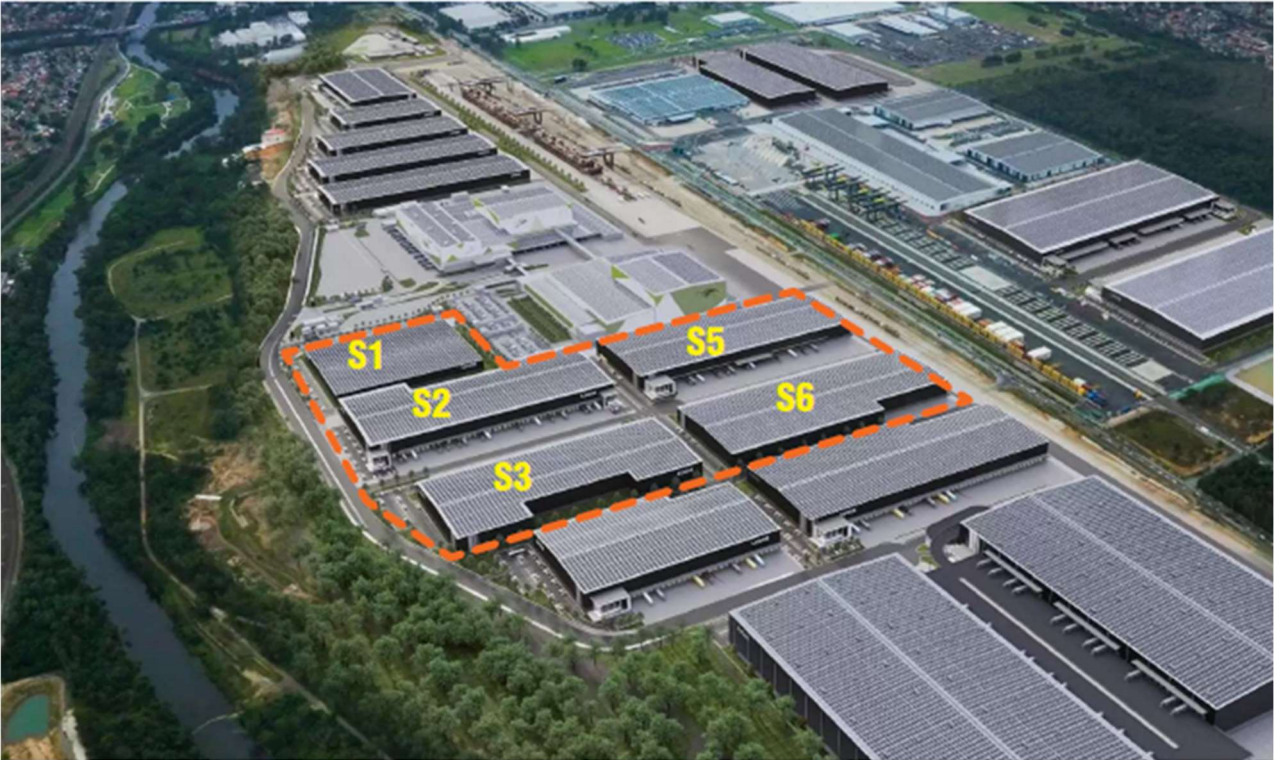
Figure 2-2 Aerial view of Warehouses S1, S2, S3, S5 and S6 (LOGOS 2023)
