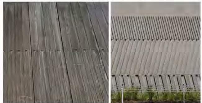
Figure 18. Retaining wall Brunswick Heads; and Noise Walls Hunter Expressway
