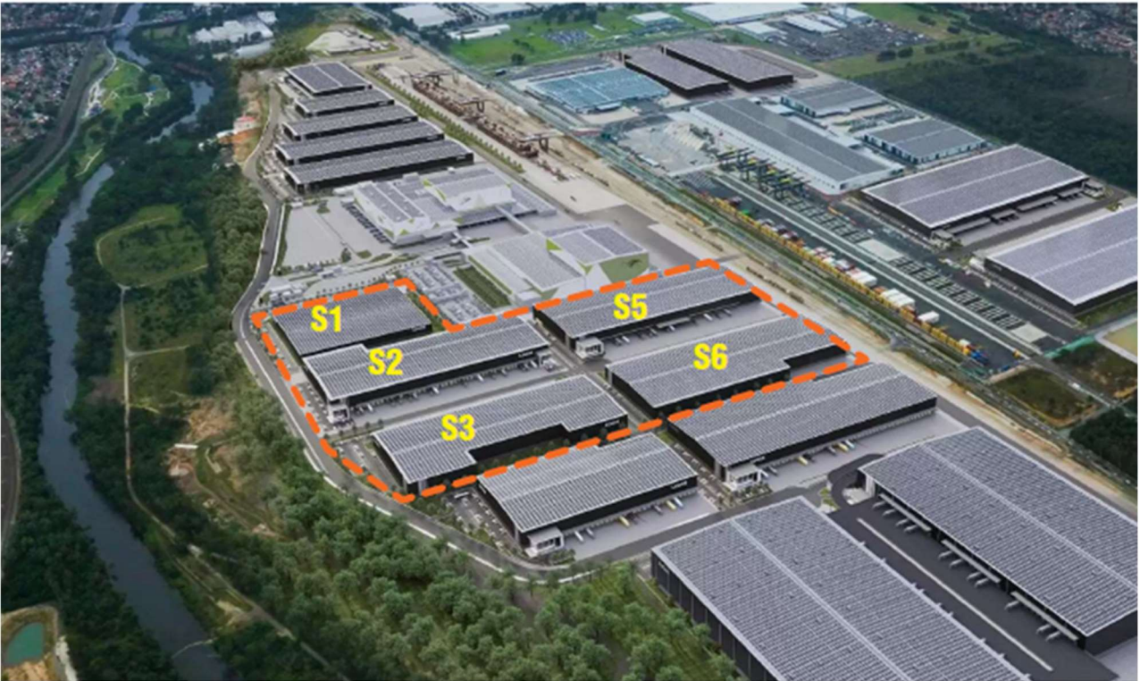
Figure 2-2 2 Aerial view of Warehouses S1, S2, S3, S5 and S6 (LOGOS 2023)
