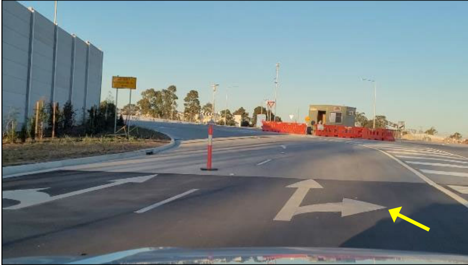
PHOTO 1: For the Western Ring Road approach to the roundabout near the BMD site office, there are two lanes on the northbound approach with only single lane exit lanes from the roundabout. Moreover, pavement markings show a through / right-turn in the median lane when there is no right-turn available.
