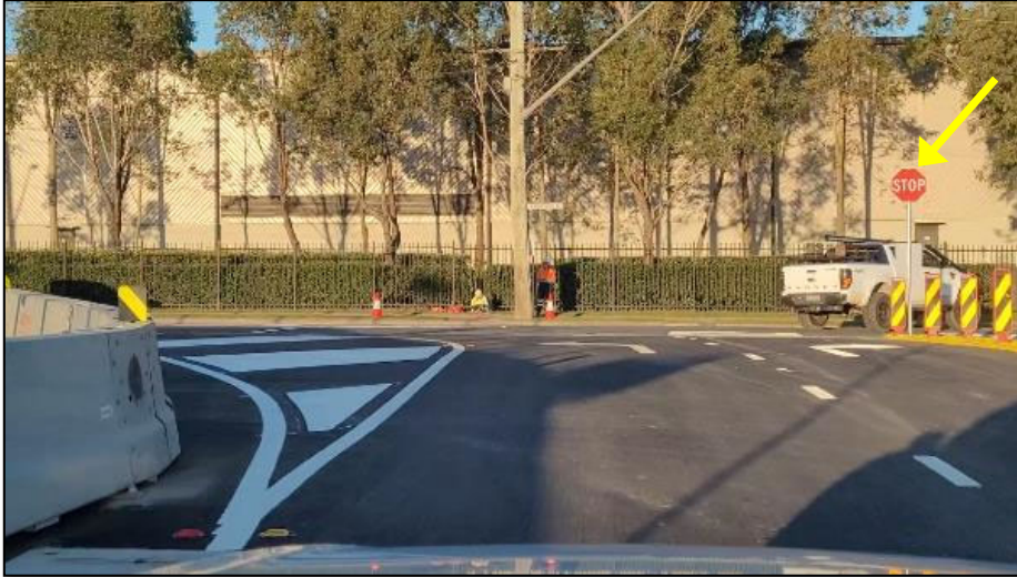
PHOTO 5: For the Bapaume Road approach to Moorebank Avenue, the 'Stop' control sign is located on the right side of the approach only, which is non-standard and undesirable, especially for the majority left-turning traffic.
