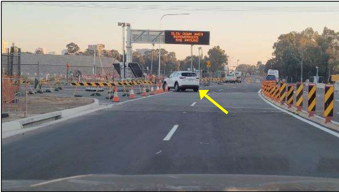
PHOTO 3: For Moorebank Avenue northbound travel, there is no physical obstruction to prevent a left-turn movement into Bapaume Road, which is a one-way exit only. During the site inspections, vehicles were observed entering Bapaume Road, ie. turning left from Moorebank Avenue northbound.
