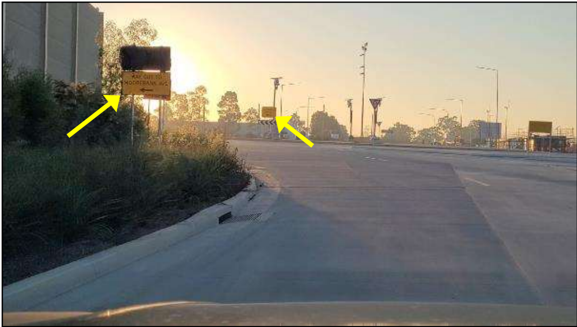
PHOTO 9: Temporary directional signage for eastbound travel along the Loop Road approaching and at the roundabout still indicates the precinct exit is via Bapaume Road, which is now incorrect.
