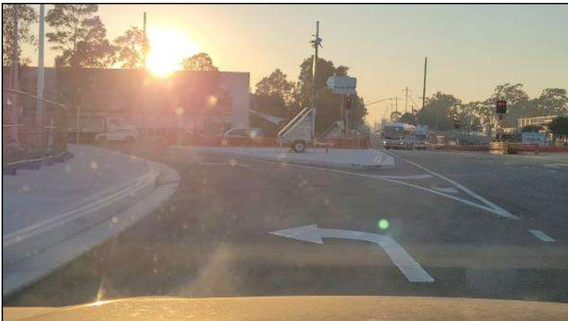
PHOTO 6: The issue of sun-glare during sunrise is applicable for eastbound travel along Bushmaster Avenue approaching the Moorebank Avenue intersection. Consequently, advisory / information signage and traffic control devices may be difficult to sight due to sun glare.
