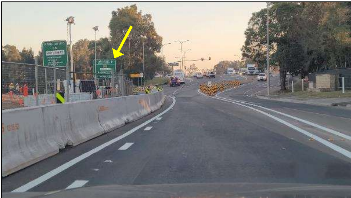
PHOTOS 7 & 8: Existing directional signage is difficult to sight / read for westbound travel along Bushmaster Avenue approaching the precinct roundabout (top photo) as well as along Moorebank Avenue northbound near the northern extent of the project works area (bottom photo).
