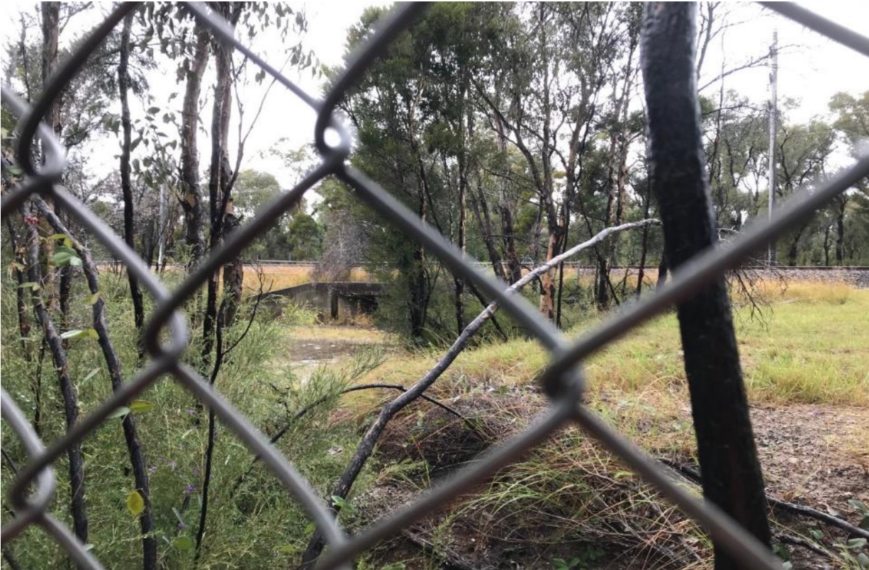
Photograph 5: Westernmost of 5 culverts at the southern end of the Bootland
