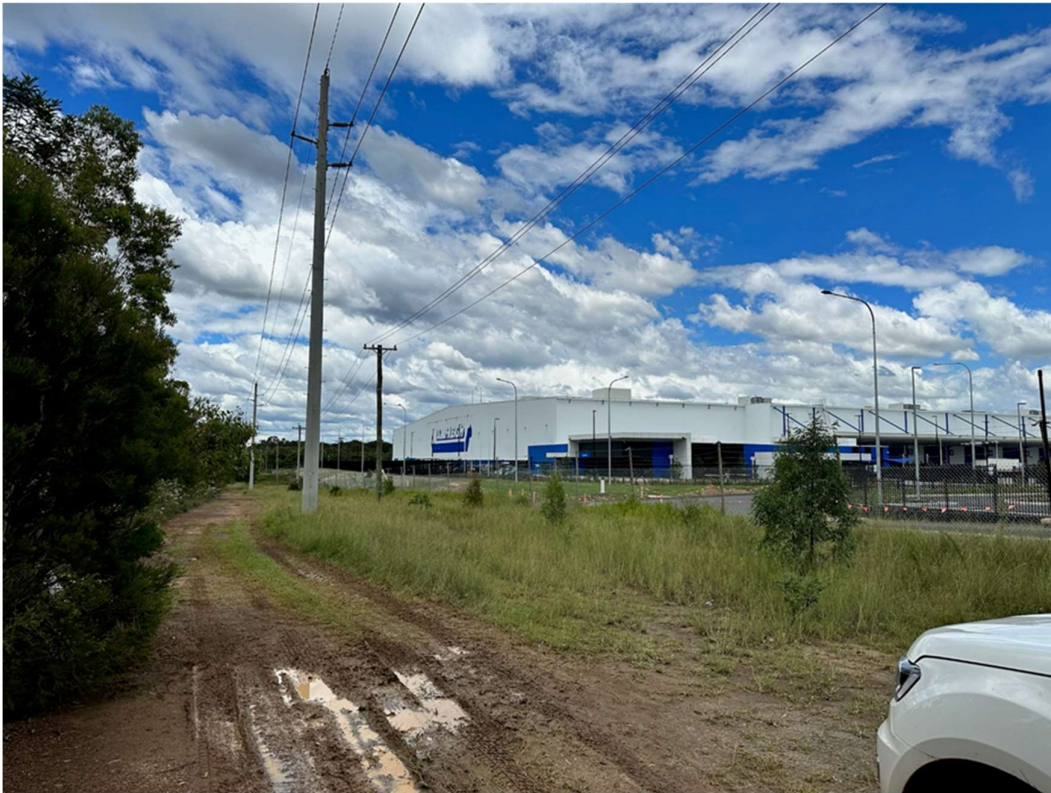
Photo 3: Project alignment and adjacent industrial area
