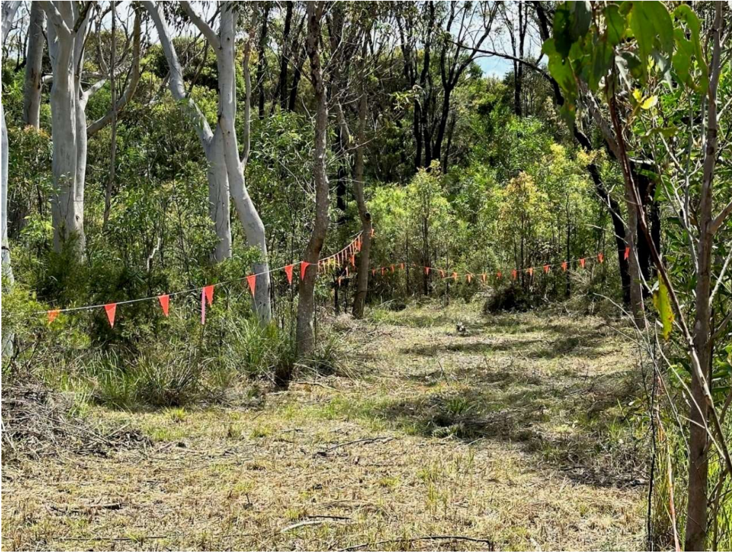
Photo 7: Cleared work area and work area boundary fencing
