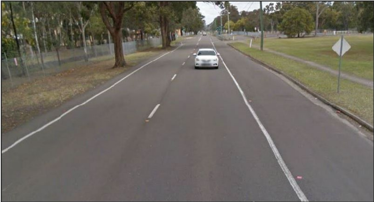
Figure 4-2: Sealed & marked road shoulders on Moorebank Avenue – permitted for on-street cycling
