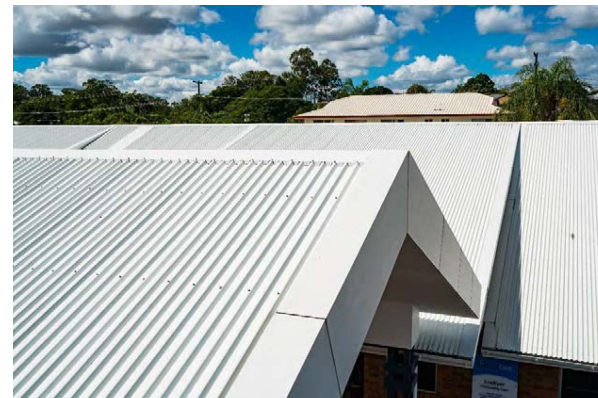
Image Source: Bluescope Colorbond Coolmax Roofing product, Albedo 0.77
