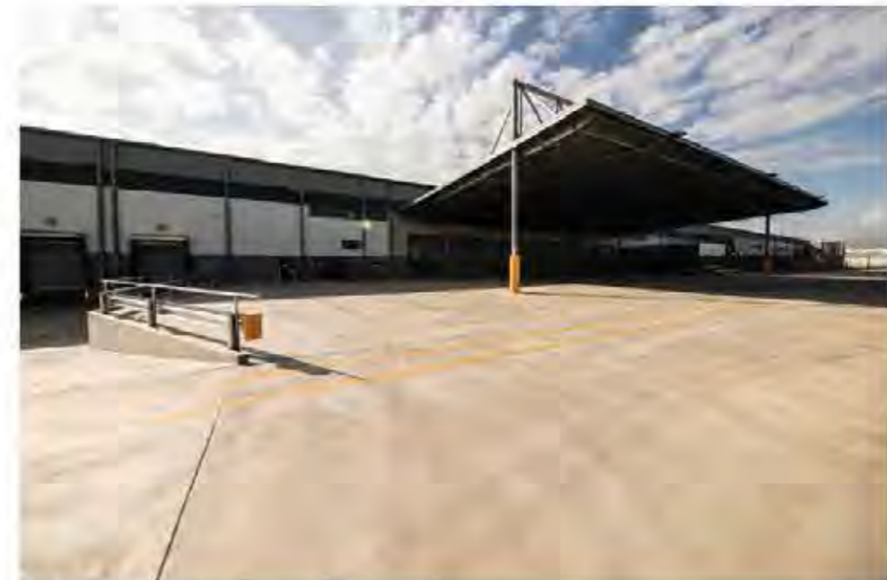
FIGURE 2.9 - Example of a South facing dock and large awning for shading at development East Warehouse 1.
