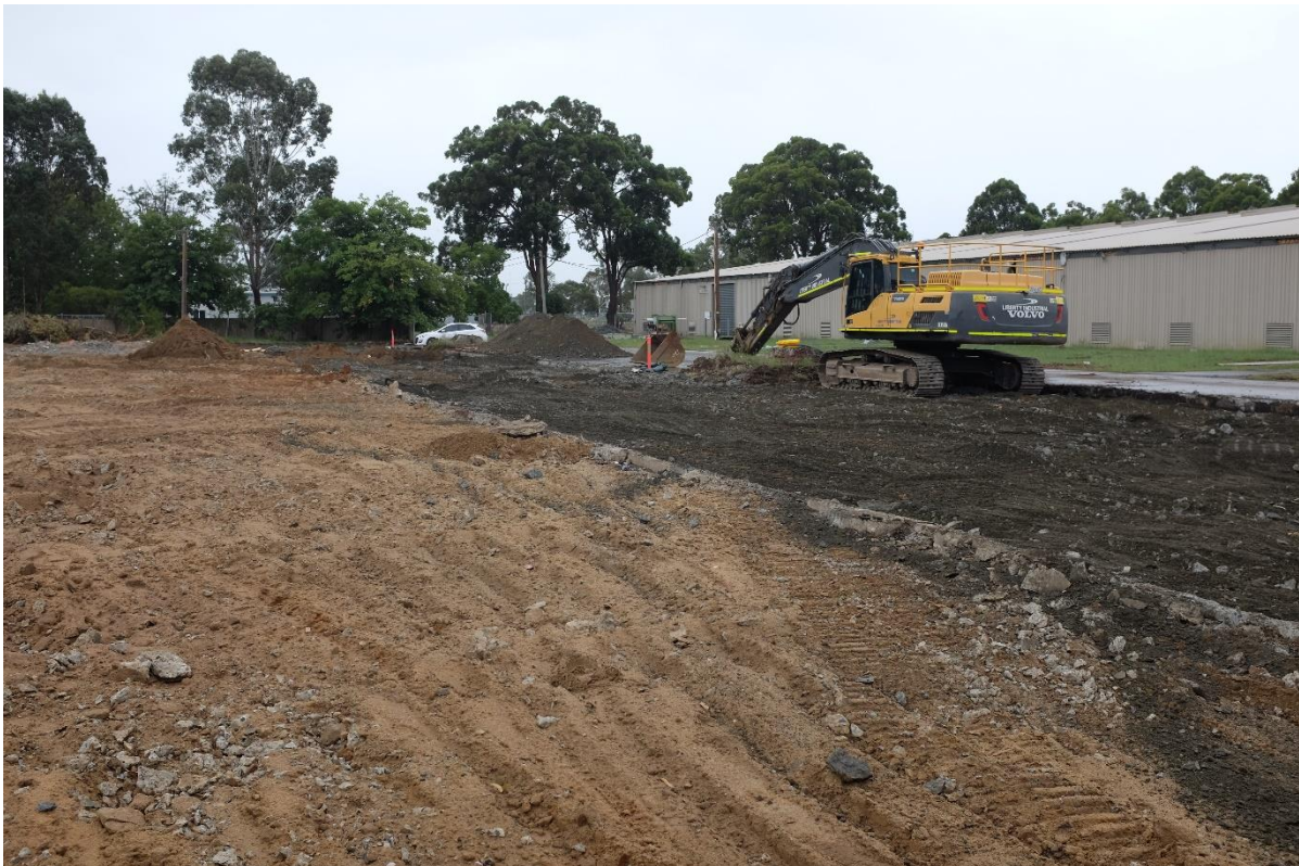
Figure 18. PAD W after slab removal and archaeological monitoring and testing. The lighter soil deposit to the left represents fill below the Warehouse 80 concrete slab (outside of PAD W). Darker soil deposits to the right represent fill below the adjoining roadway and associated concrete slabs (PAD W). View northeast towards PAD V.
