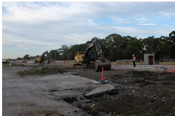
Figure 15. PAD W during slab removal monitoring works, view southwest.
