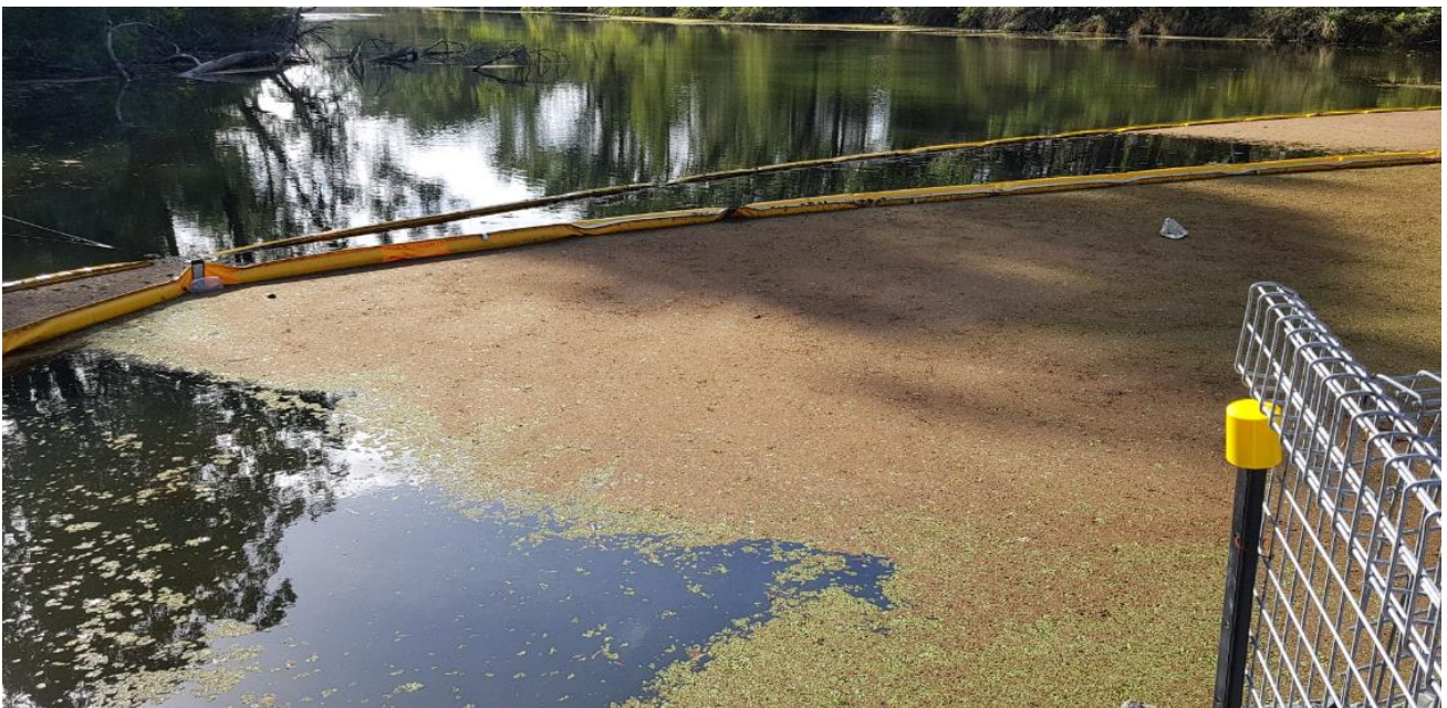
Plate 2: Silt curtains in Georges River.
