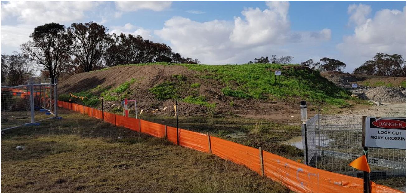
Plate 7: Stabilised stockpile.
