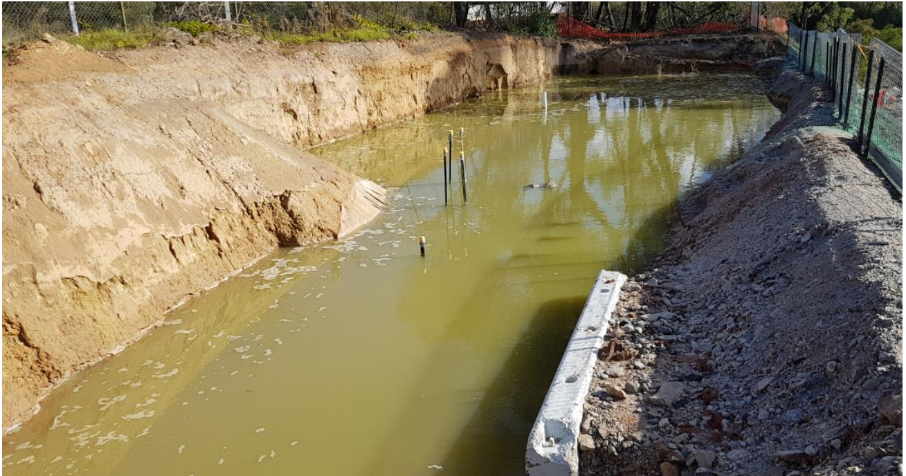
Plate 5: Sediment basin following rain (recorded overnight prior to site visit).
