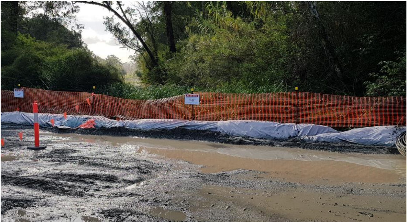
Plate 1: Boundary control and erosion and sediment control.
