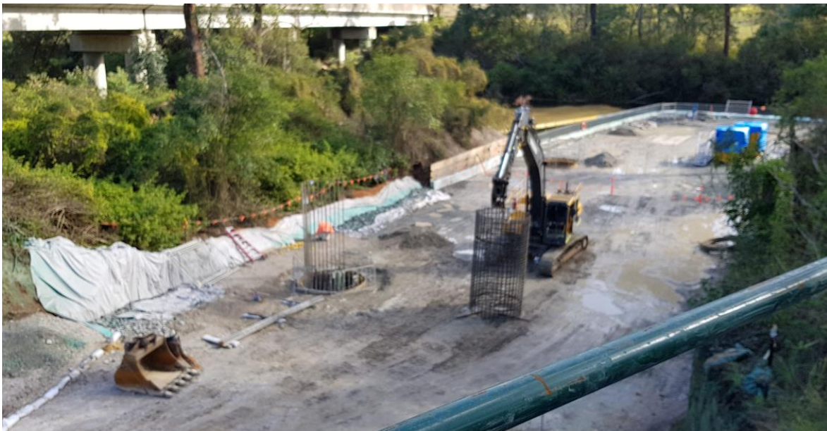
Plate 4: Georges River works overview, with boundary flora and fauna controls and erosion and sediment controls in place.
