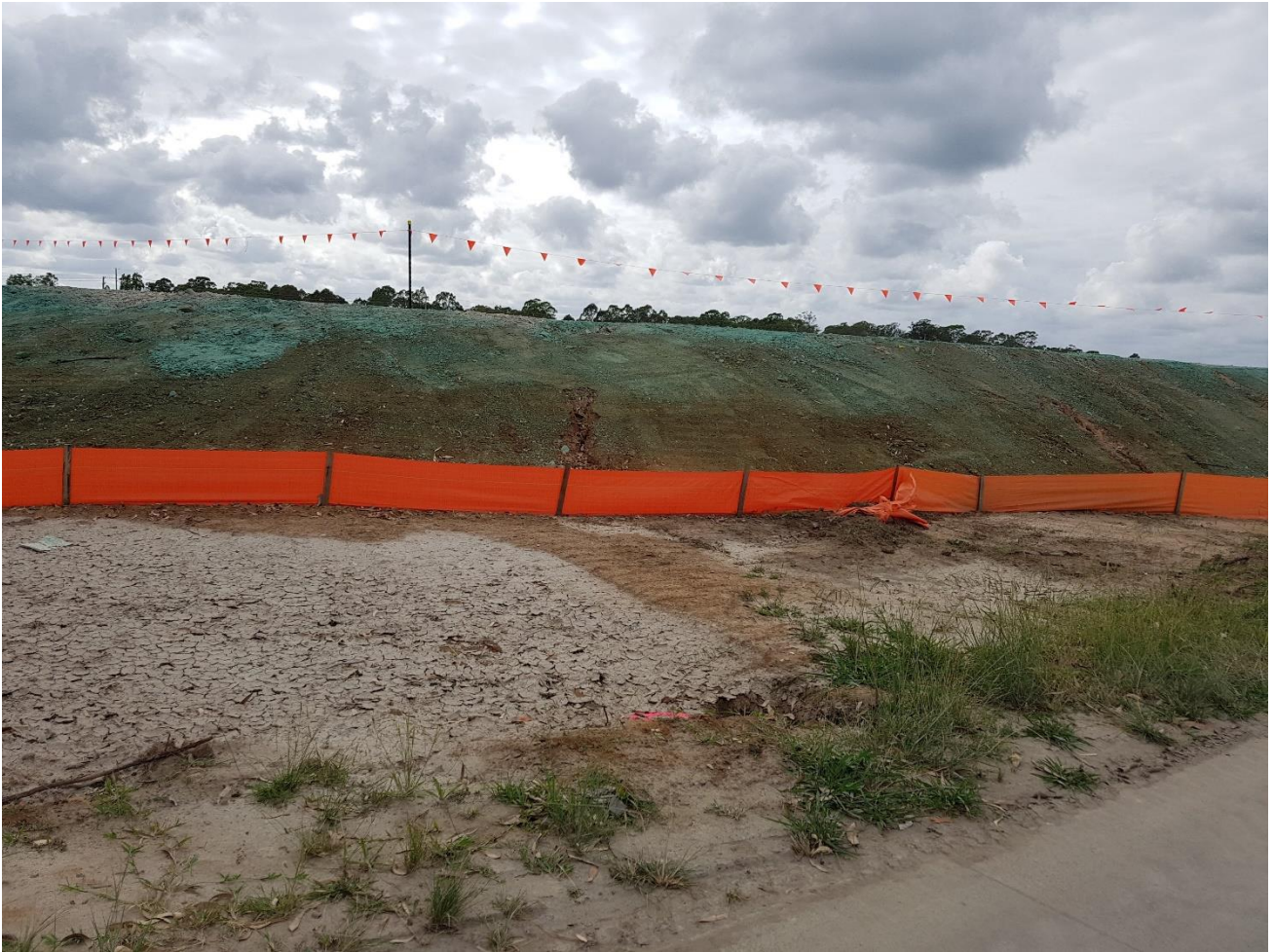
Plate 6: Silt fencing and polymer coating of batter slope.
