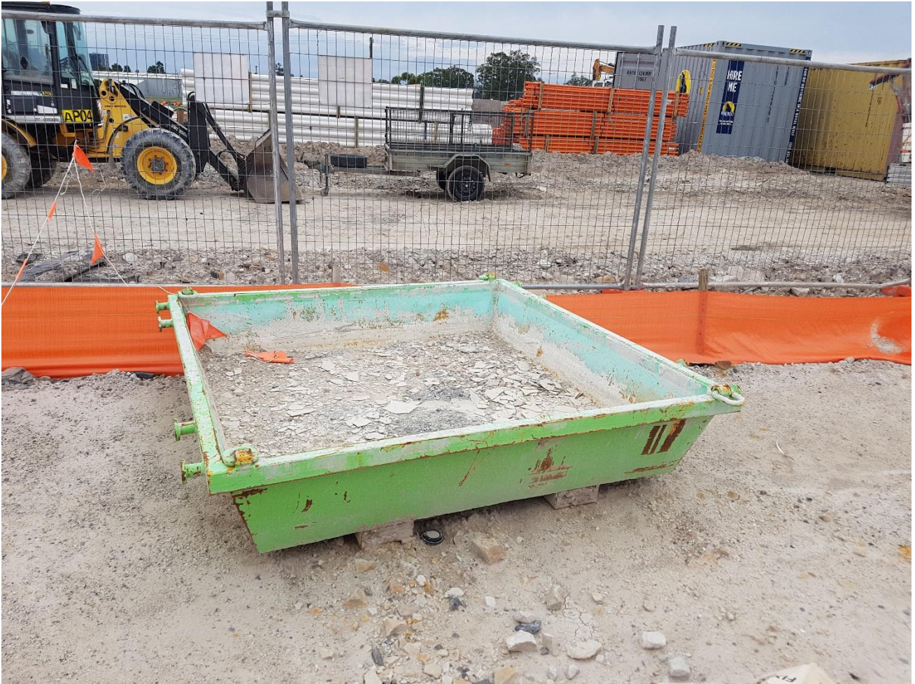
Plate 7: Concrete washout tray.
