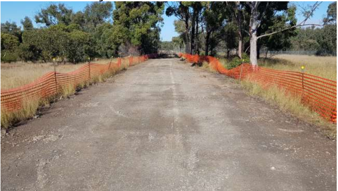
Photo 2: Remedial works on disused rail spur
