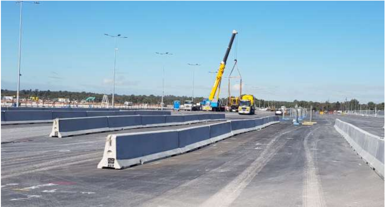
Photo 7: rail connection with track grinder delivery underway
