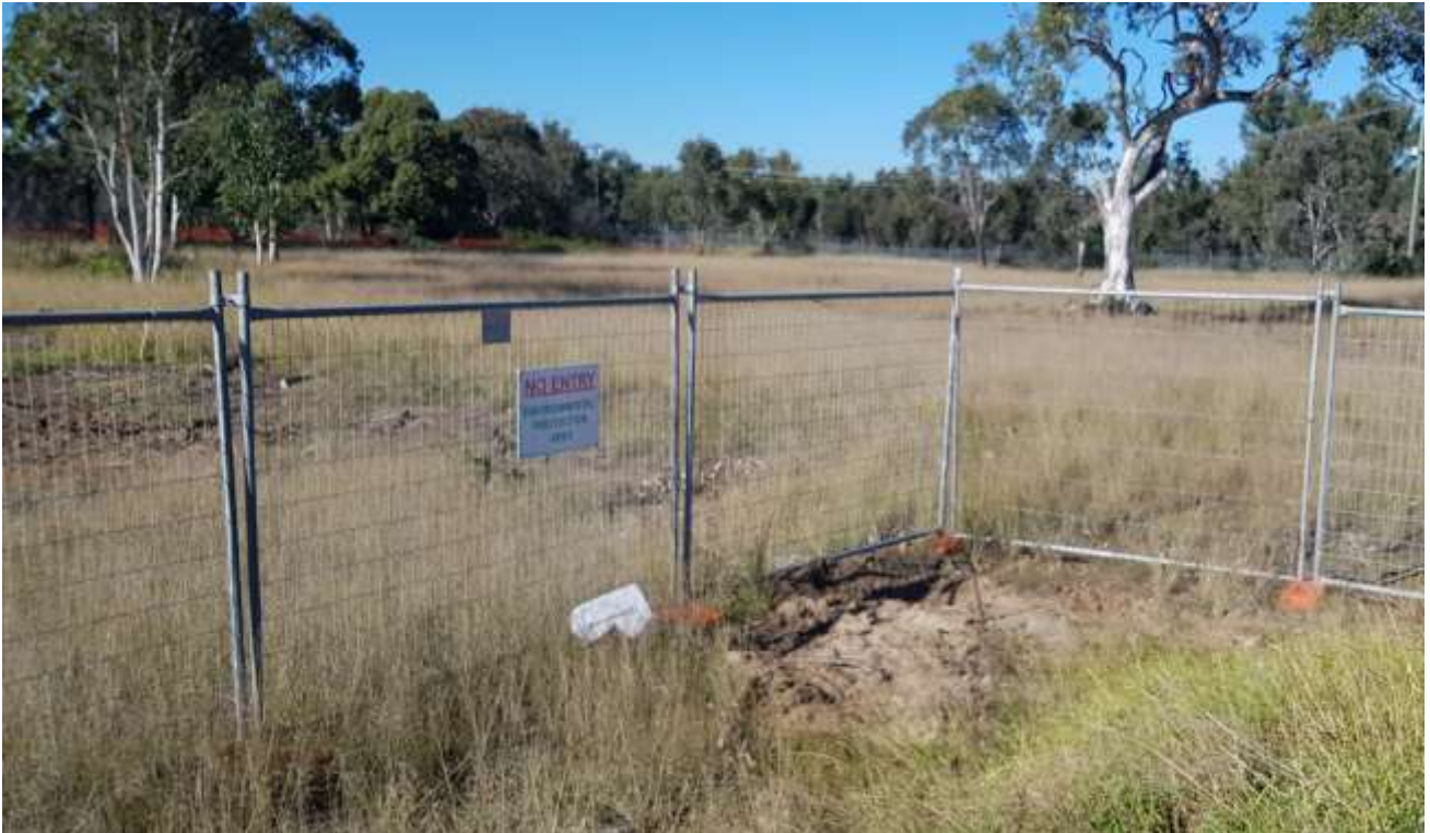
Photo 1: Environmental no-go demarcation
