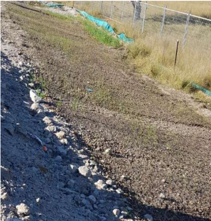
Photo 6: batter stabilization through revegetation
