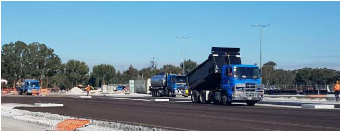
Photo 5: surface works ongoing
