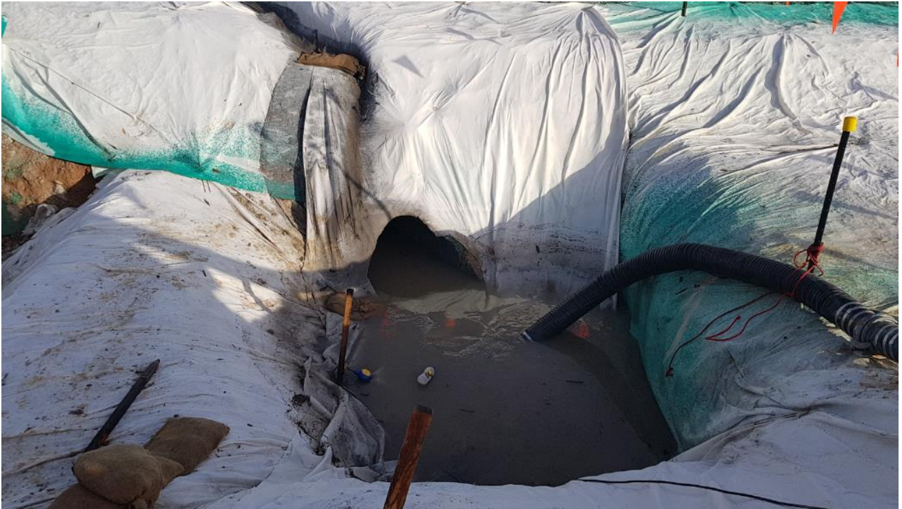
Plate 5: Pump out of basin to watercart.
