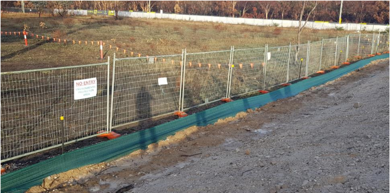
Plate 1: Boundary sediment control, fencing and environment protection zone signage.
