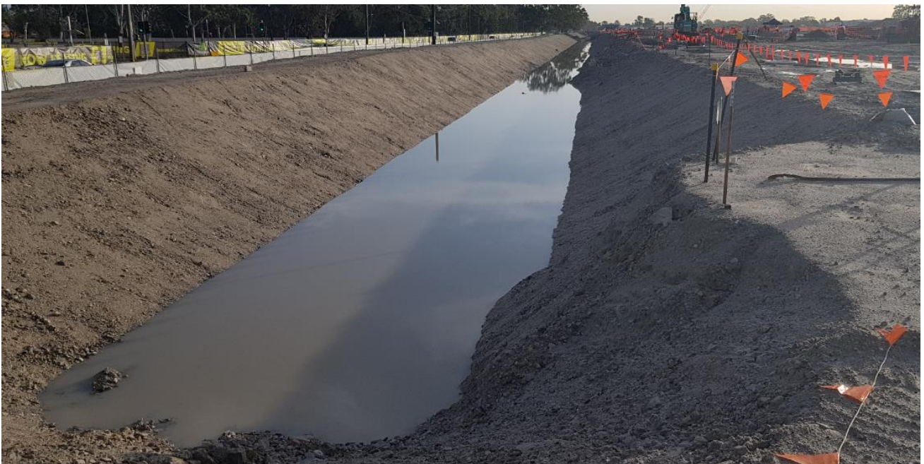
Plate 2: Swale drain / basin capturing runoff from overnight rainfall.
