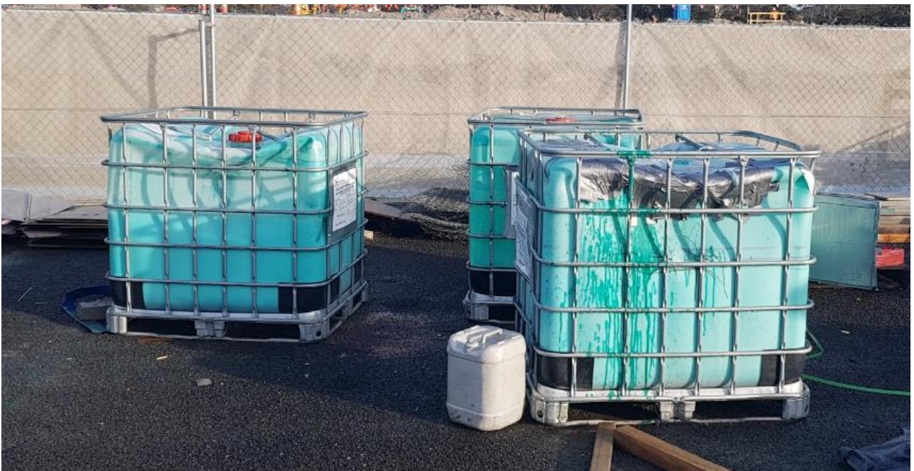
Plate 4: Dust suppression polymer on hardstand.
