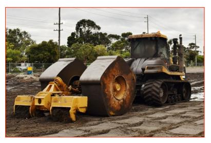
Undulations are created during the impact compaction. To enable the impact compactor to travel at operating speed a scraper attachment is fitted to the impact compactor. If the undulations become excessive the operator shall engage the scarper attachment to trim the undulations.
