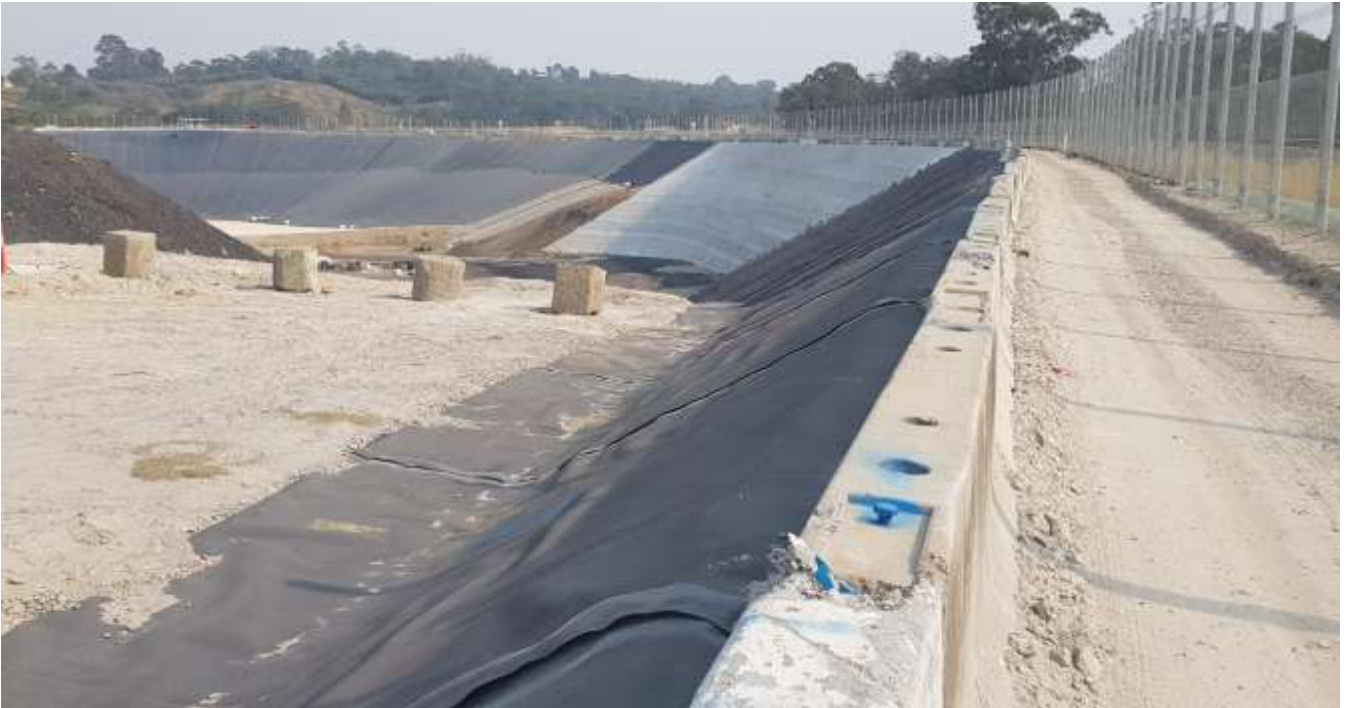
Figure 2: The rail formation and Gelinfeld Waste Facility cell.
