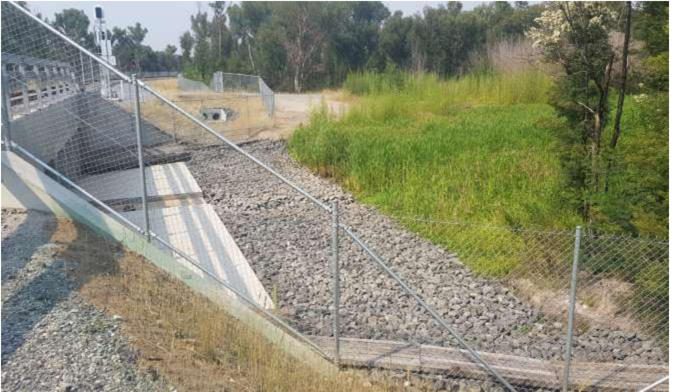
Figure 7: Anzac Creek crossing with scour protection.
