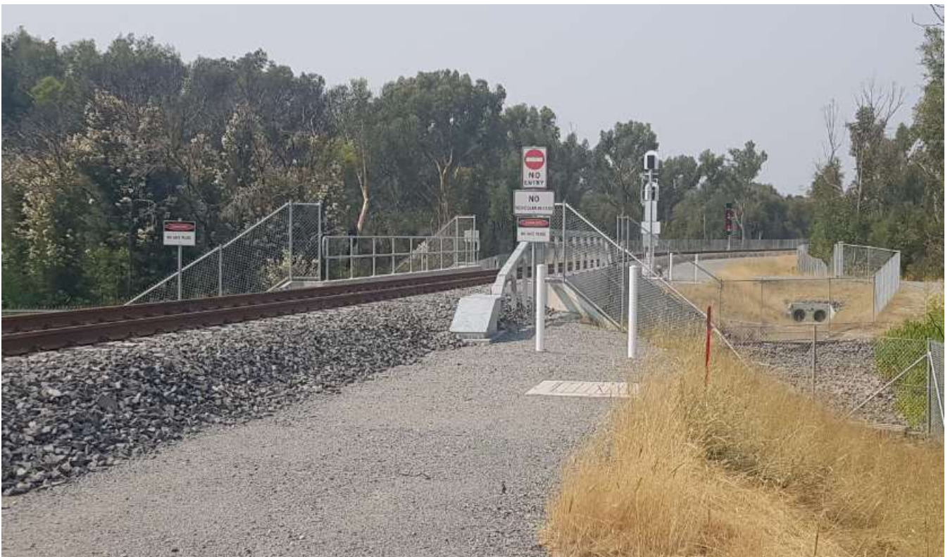
Figure 6: Signalling installed at Anzac Creek.
