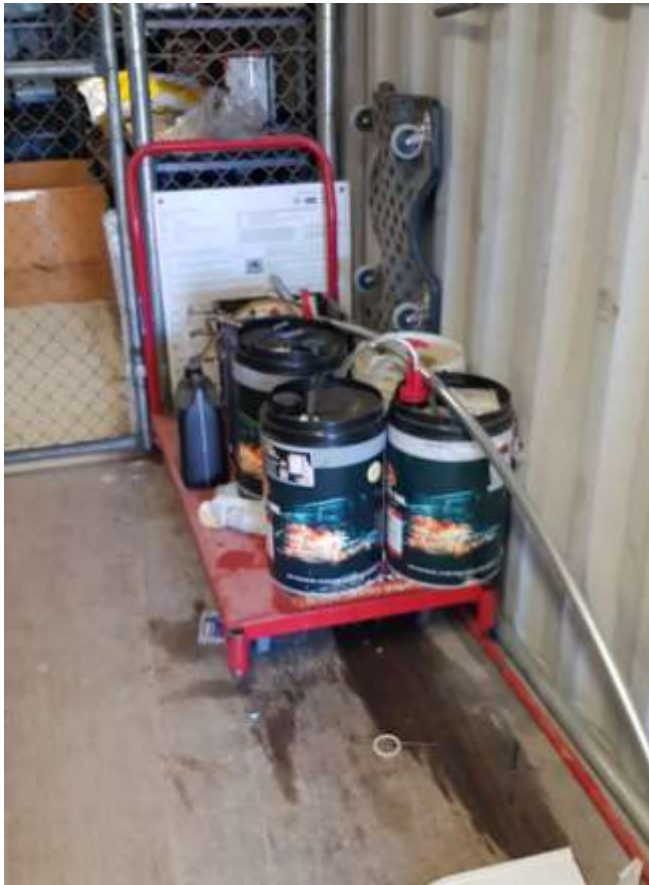
Photo 2: 40L drums at ResourceCo outside of bund.
