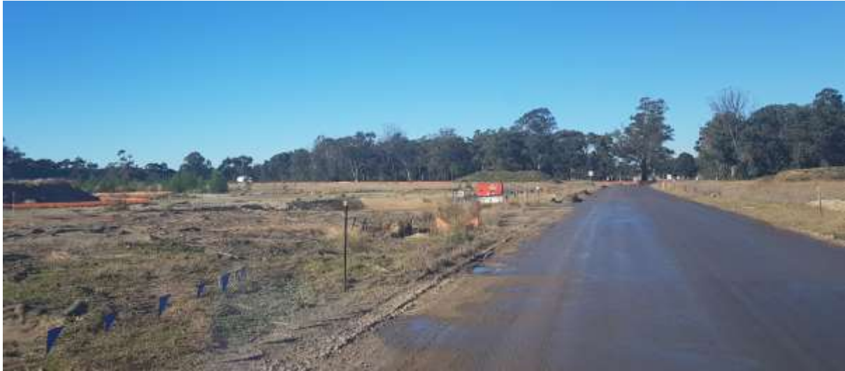
Photo 8: Dust suppression on haul roads
