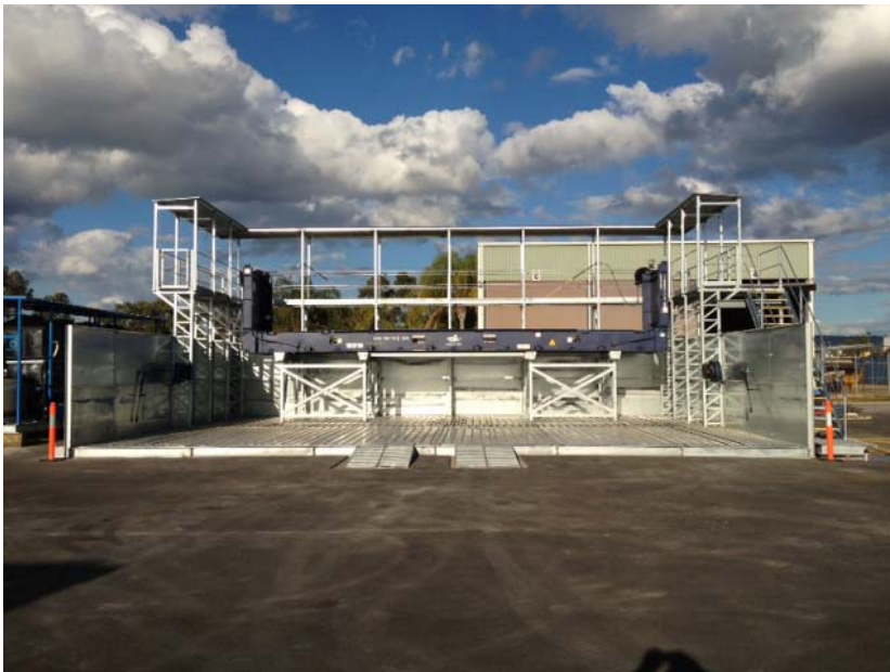
Figure 6-2: Example of a container wash-down facility and de-gassing area
