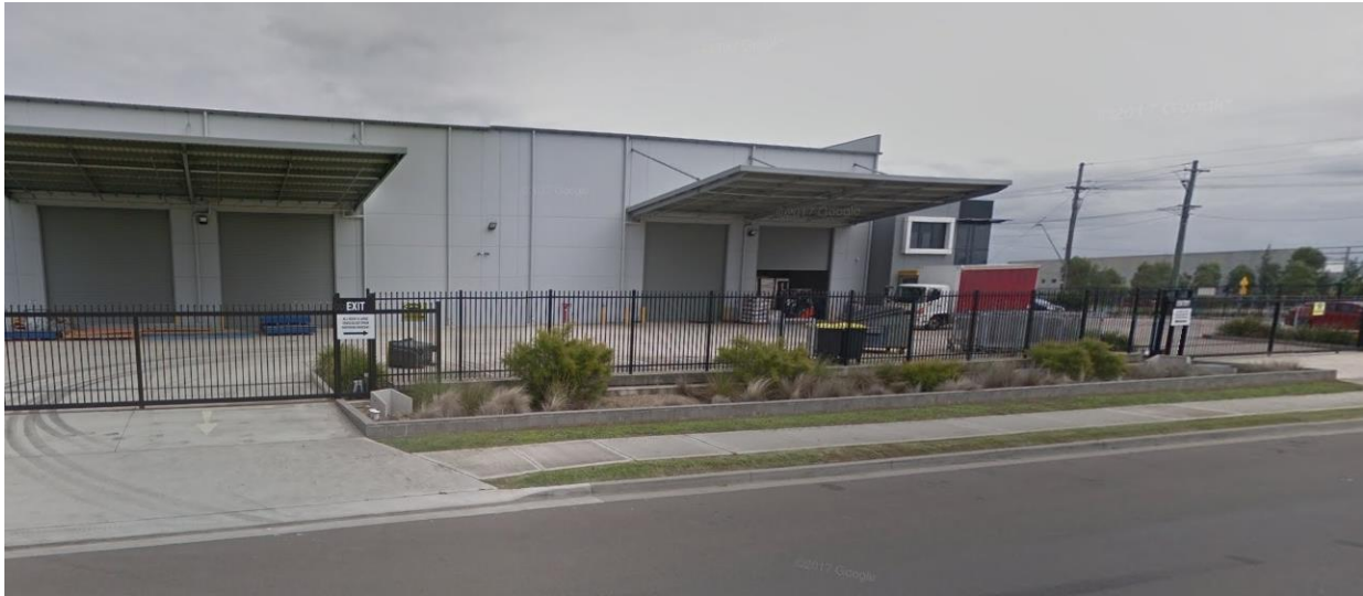
Figure 5-3: Example of bioretention system in setback area of an Industrial development.
