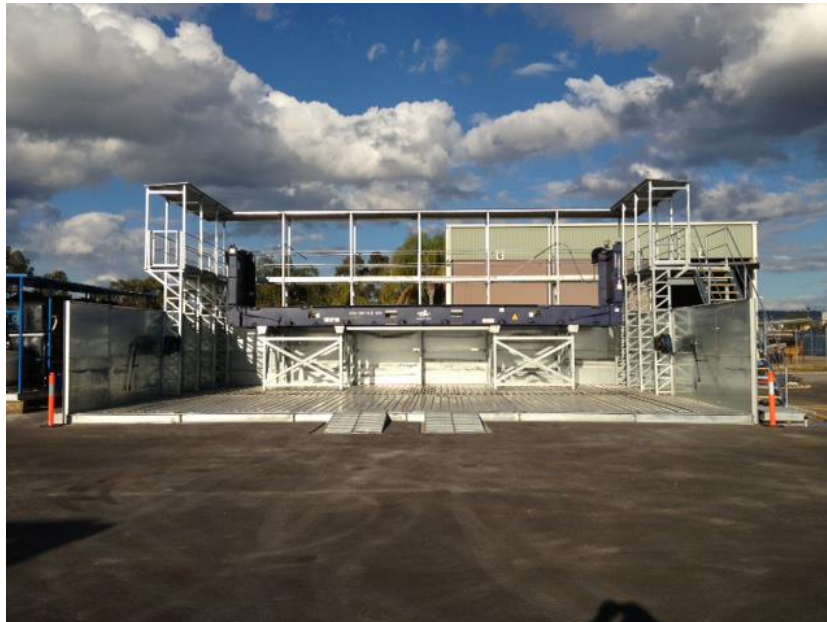
Figure 4-6: Example of a container wash-down facility and de-gassing area
