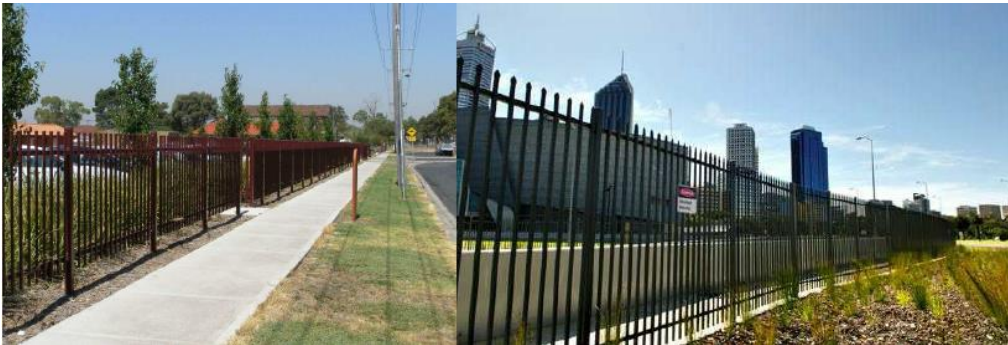
Figure 4-8: Palisade security fence example
