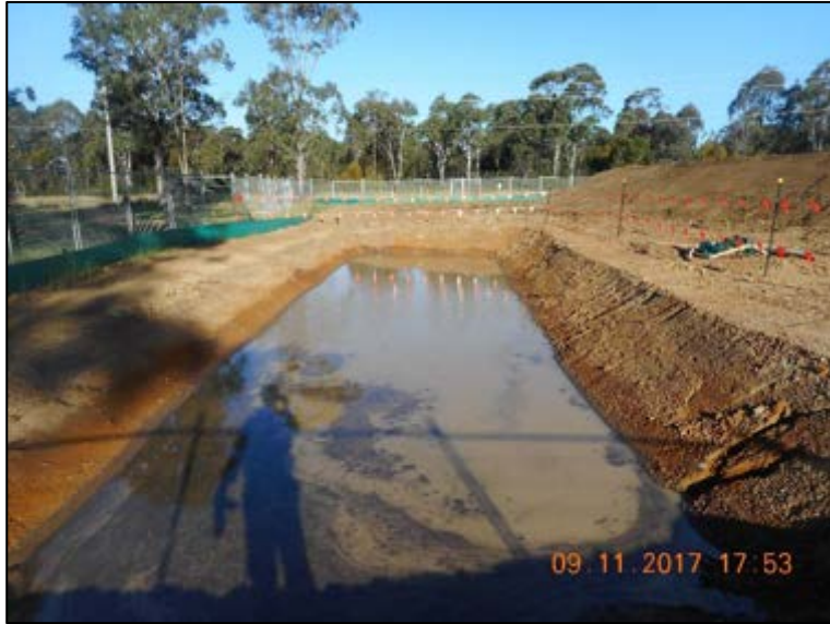
Inspecting basin for water level, and sample collection
