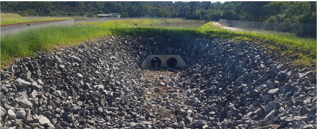
Photo 9: On Site Detention at Glenfield Waste Services.
