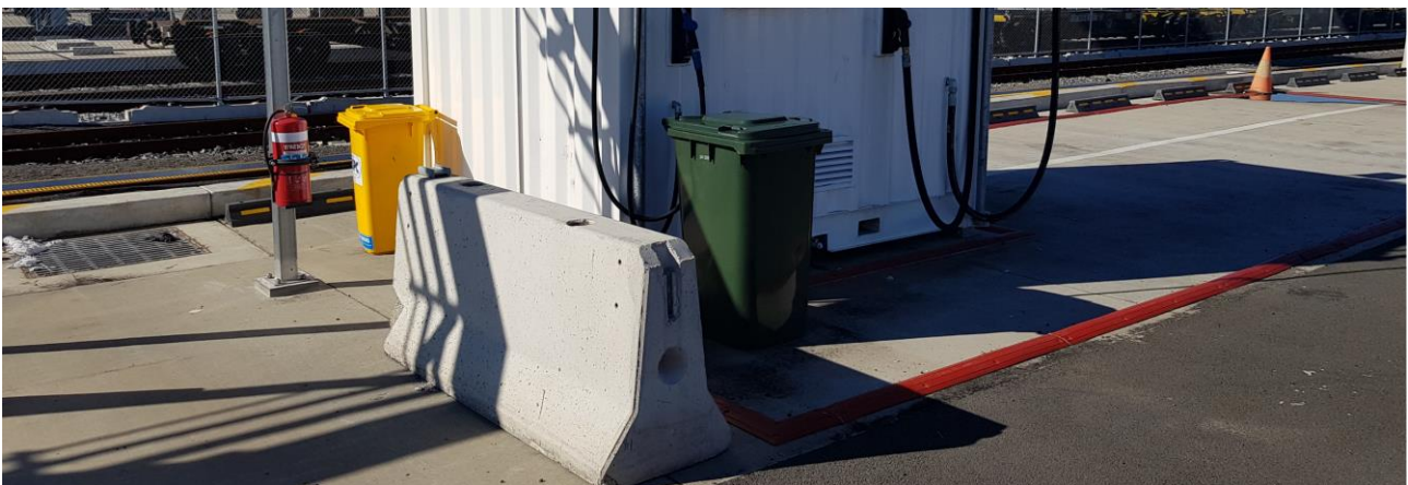
Photo 2: Inadequate bund (red barrier) at the Reach Stacker crane refuelling area. Note the Rail Link at rear and stormwater pit on left of shot.
