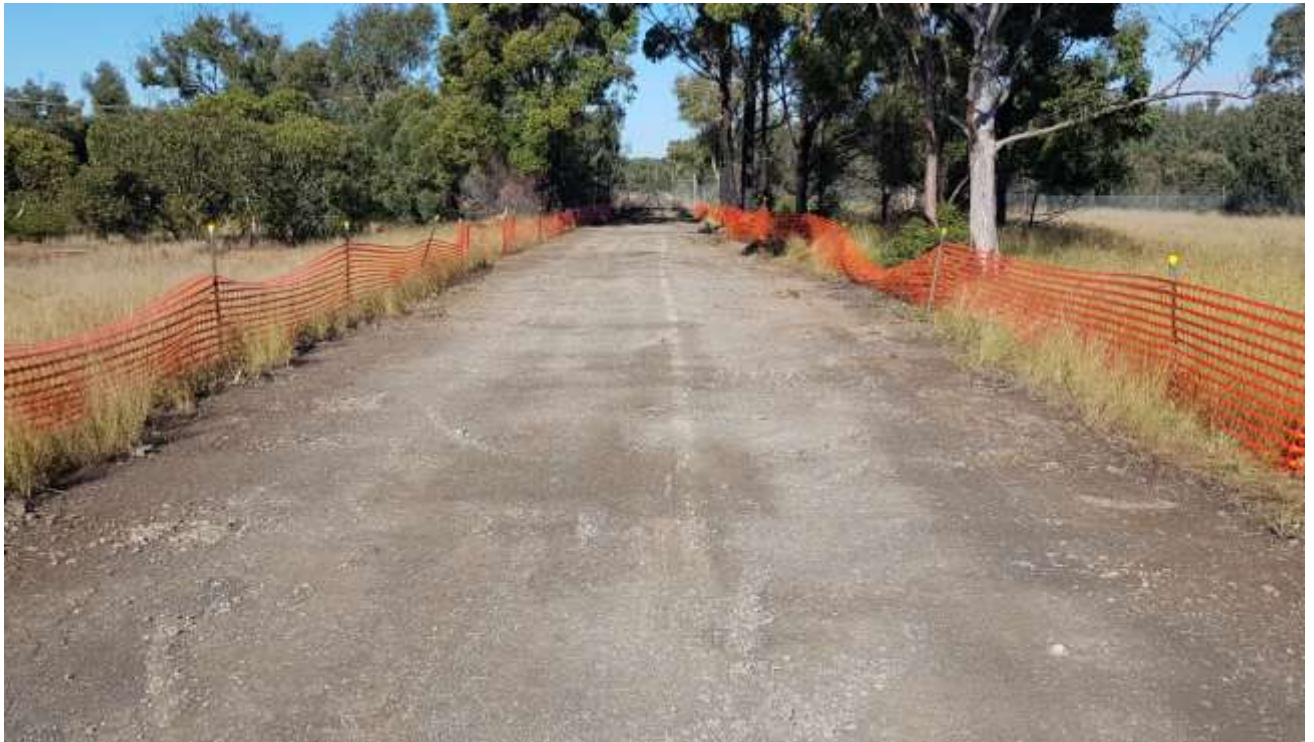
Photo 13: Remedial works on disused rail spur
