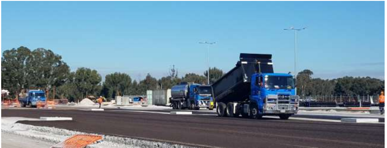
Photo 16: Surface works ongoing
