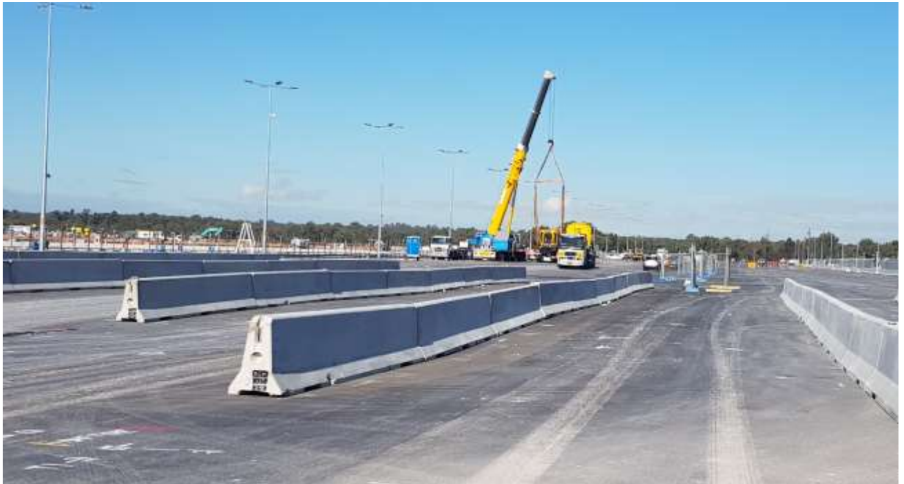
Photo 18: Rail connection with track grinder delivery underway
