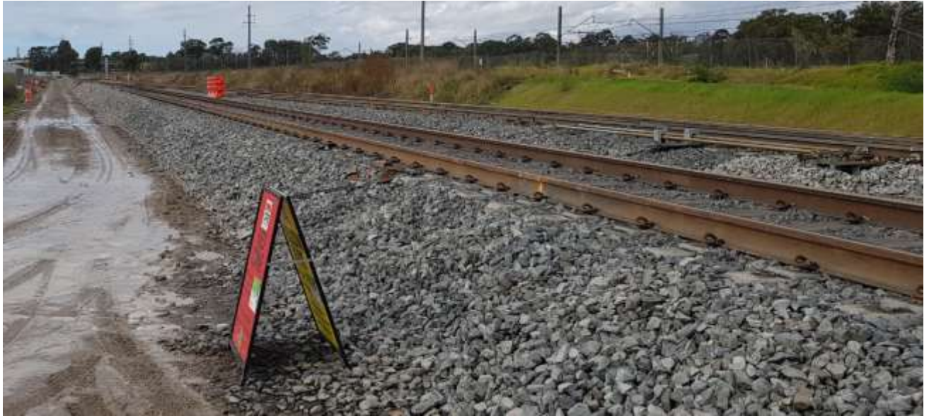
Photo 1: Track installed along majority of rail corridor.
