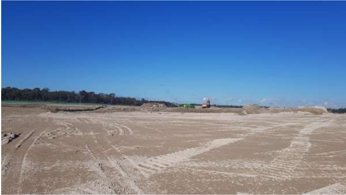
Photo 20: MPE Stg 2 bulk earthworks
