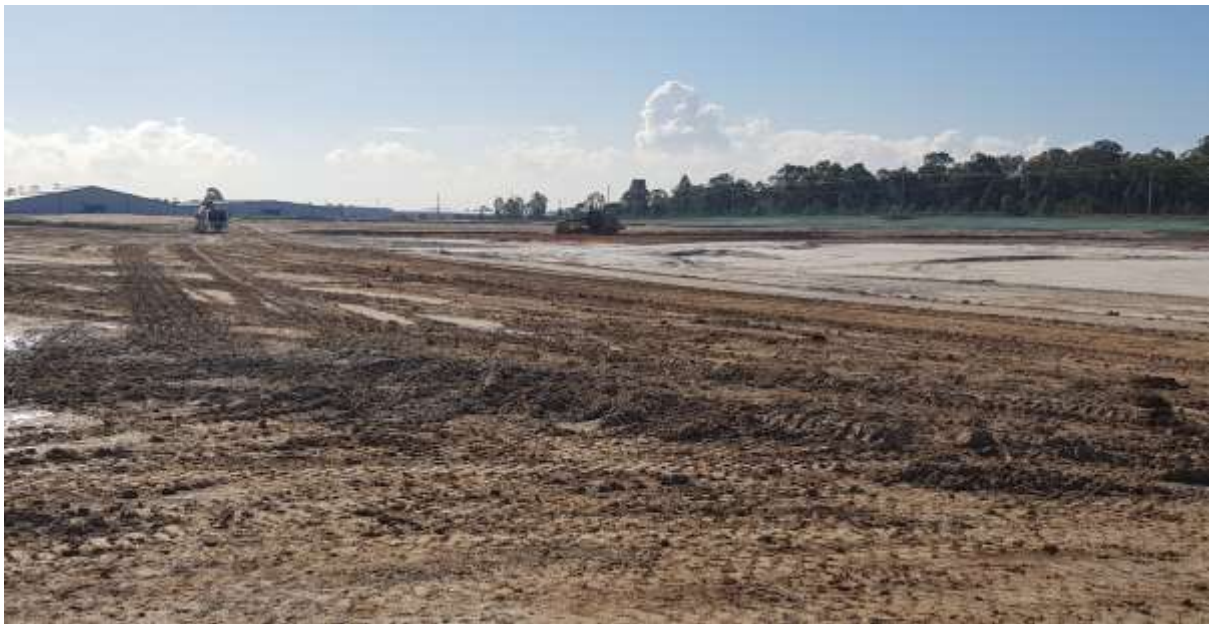
Photo 21: MPE Stg 2 bulk earthworks
