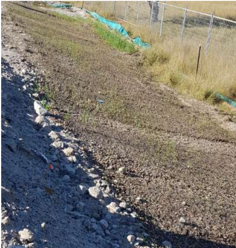
Photo 17: Batter stabilization through revegetation
