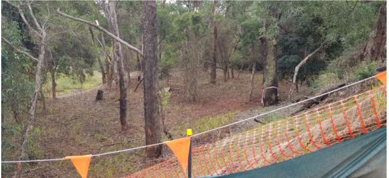
Photo 3: Weed management and revegetation at Georges River Bridge.
