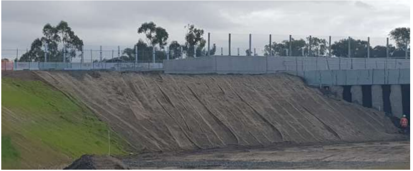
Photo 7: Site rehabilitation at Moorebank Avenue underpass.
