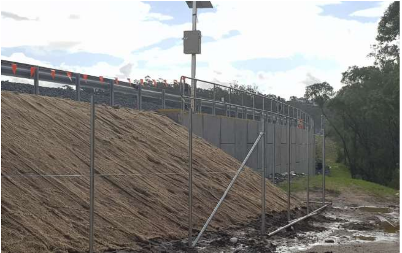
Photo 11: GWF rail alignment with rehabilitation underway
