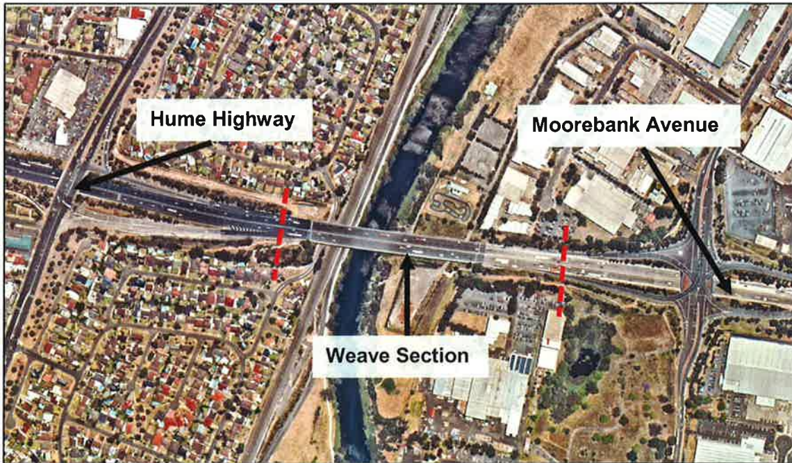
Figure 6: M5 Motorway, between Moorebank Avenue and the Hume Highway (Base Image Source: Nearmap 2015)
