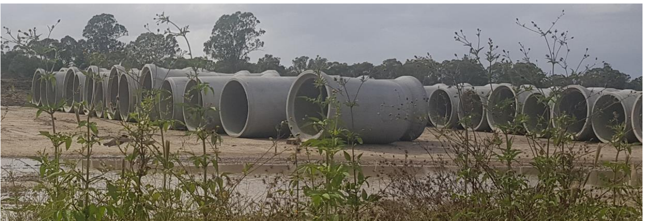
Photo 5: Drainage infrastructure in preparation for install
