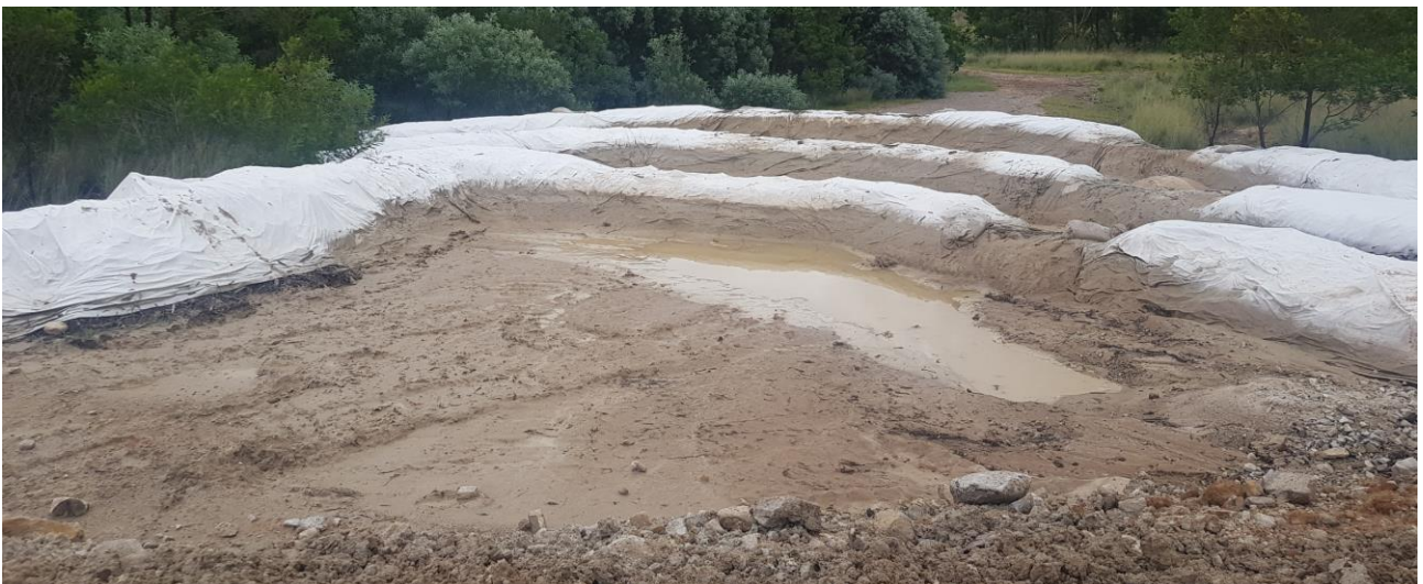
Photo 9: Erosion and sediment controls.
