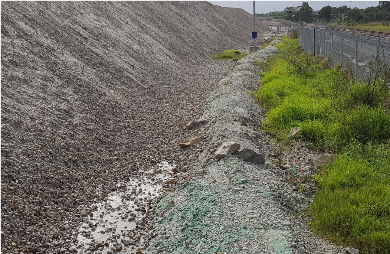
Photo 6: erosion and sediment control
