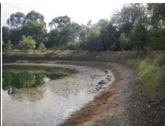
Plate 54. Leachate dam in Glenfield Waste Facility
