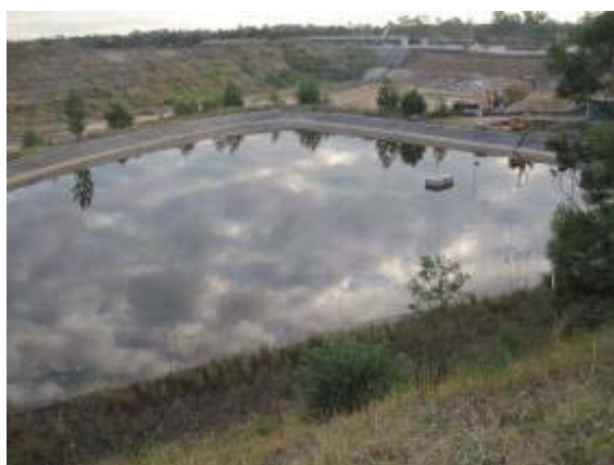
Plate 53. Dam in Glenfield Waste Facility
