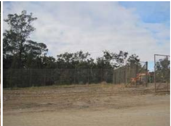
Plate 58. Glenfield Waste Facility is bound by chain-mesh fencing
