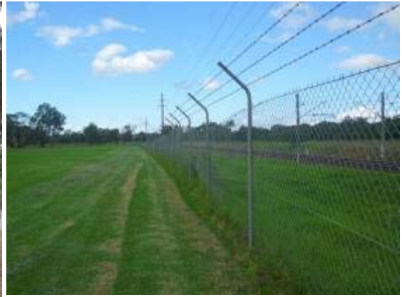
Plate 56. Rail Corridor bound by chain mesh fencing adjoining East Hills Rail Line
