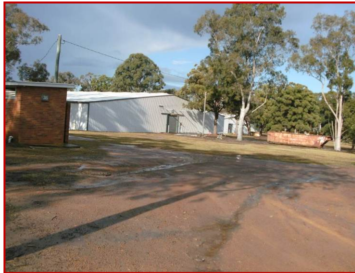
Figure 12. An example of development within the SIMTA site. This structure is located in the south and east of the SIMTA site and the exposures in the foreground represent a mixture of natural truncated B horizon and introduced fill. The trees in the background, despite their size, were planted in the 1950s.
