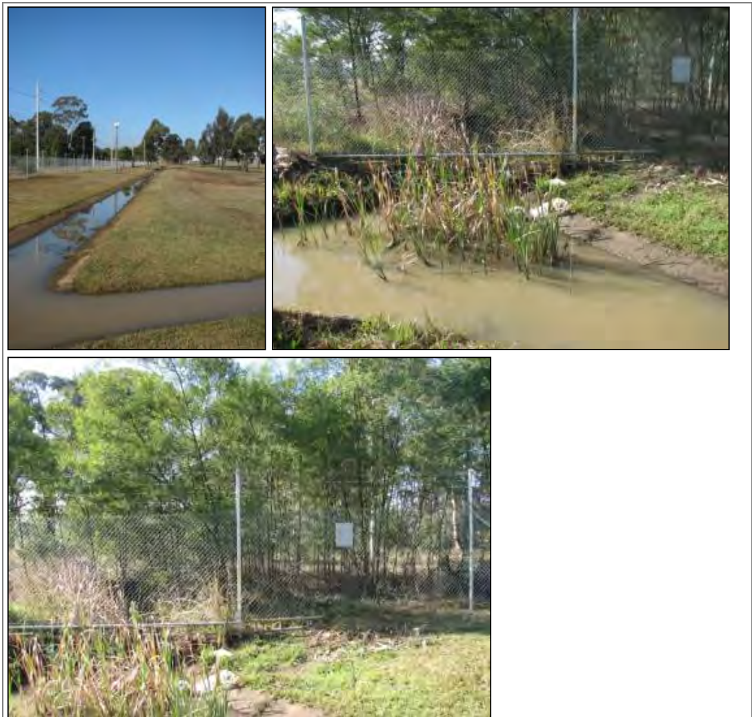
Photos show channelled approaches and piped crossing under Greenhills Avenue from the northern outlet point
