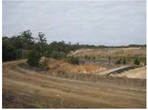
Plate 40. Glenfield Waste Disposal site
