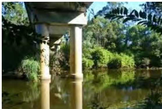
Plate 44. Georges River beneath rail bridge
