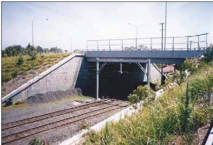
Figure 7 – Overbridge with Reinforced Soil Walls at Abutments
