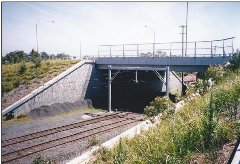
Figure 7 – Overbridge with Reinforced Soil Walls at Abutments
