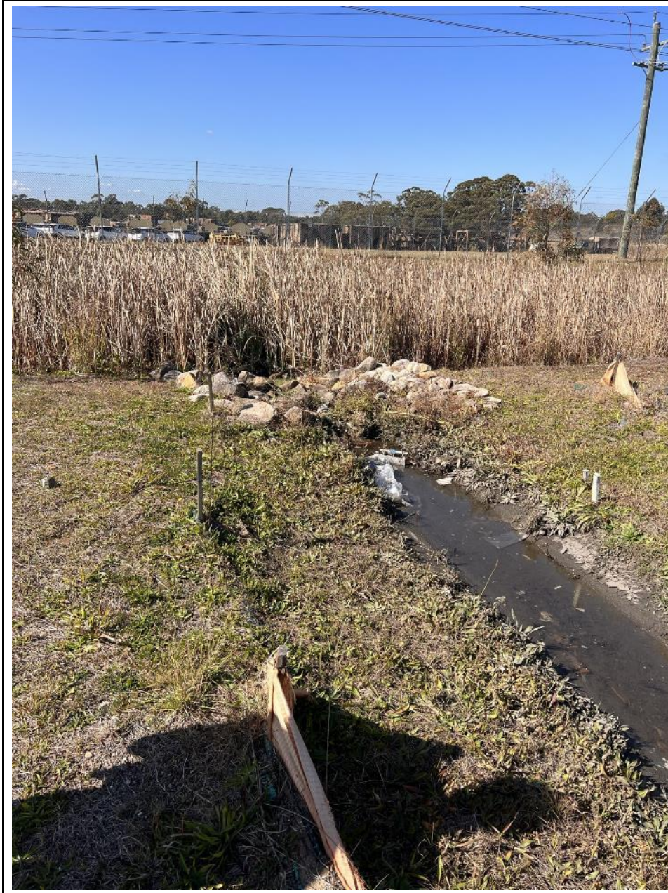
Photo showing some litter present prior to discharge into Swale 1. This is from an untreated part of the existing development which is yet to be developed.
