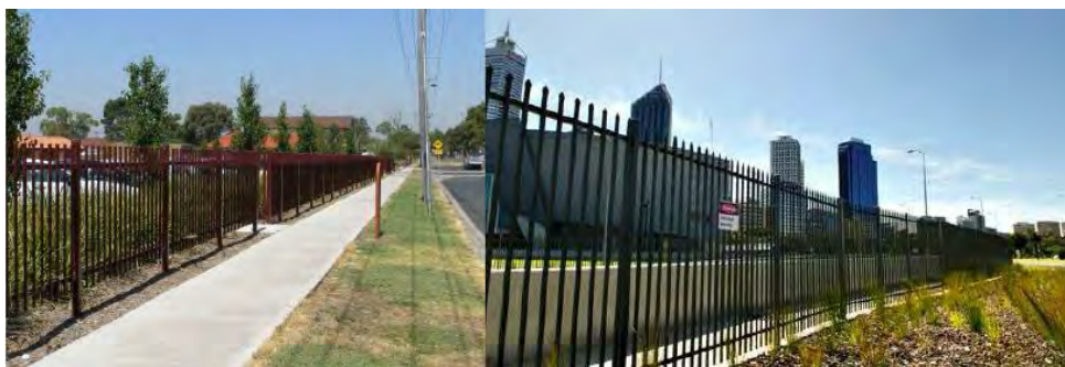
Figure 4-7 Palisade security fence example
