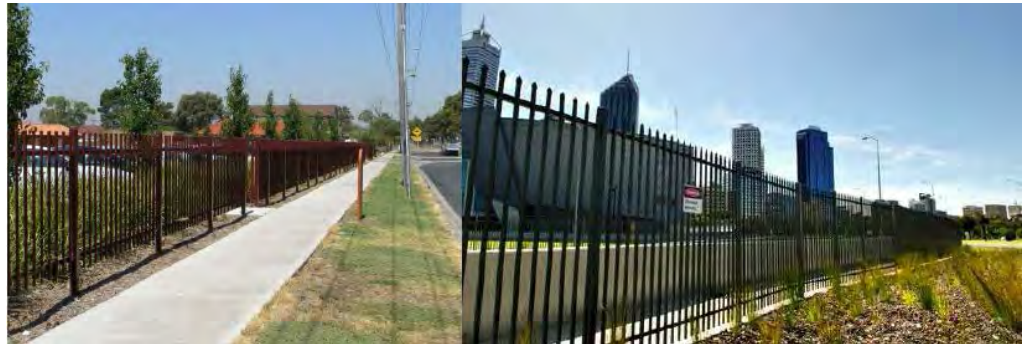
Figure 4-7: Palisade security fence example
