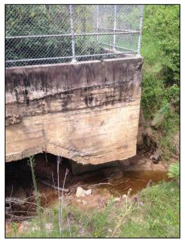
Photo 5-5: Channel failure and viewing viewing south-west
