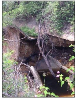
Photo 5-2: Channel failure and scouring viewing upstream (eastward)
