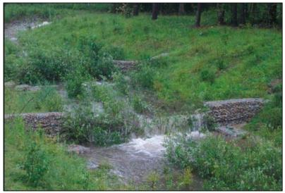
Photo 5-6: Vegetated gabion structures
