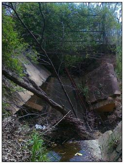
Photo 5-3: Channel failure and scouring viewing downstream (westward)
